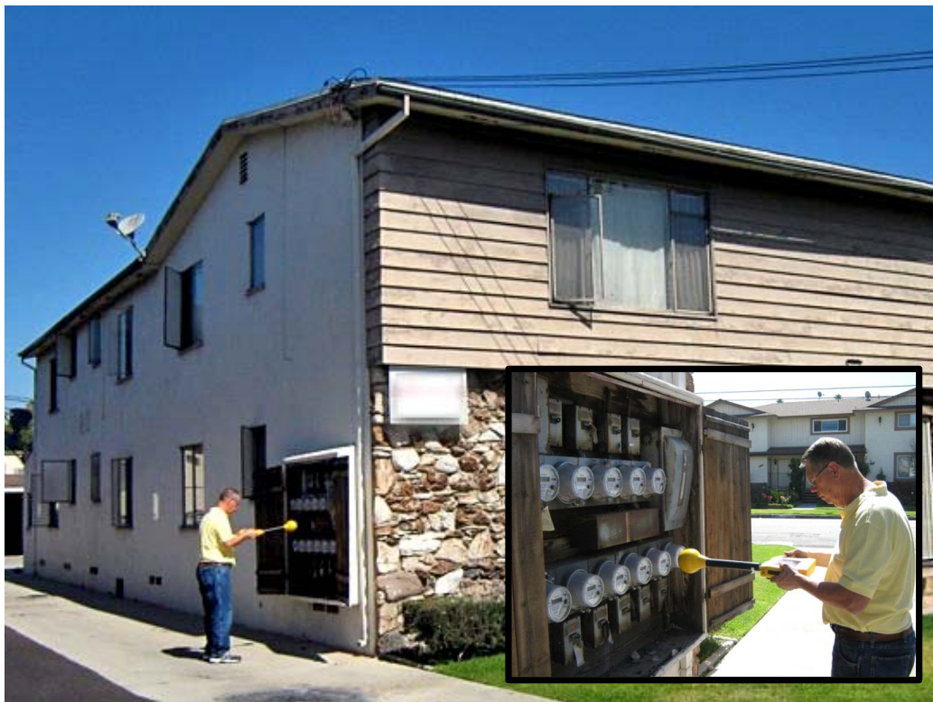
Figure 7 Measuring RF power densities in front of an outdoor bank of smart meters
