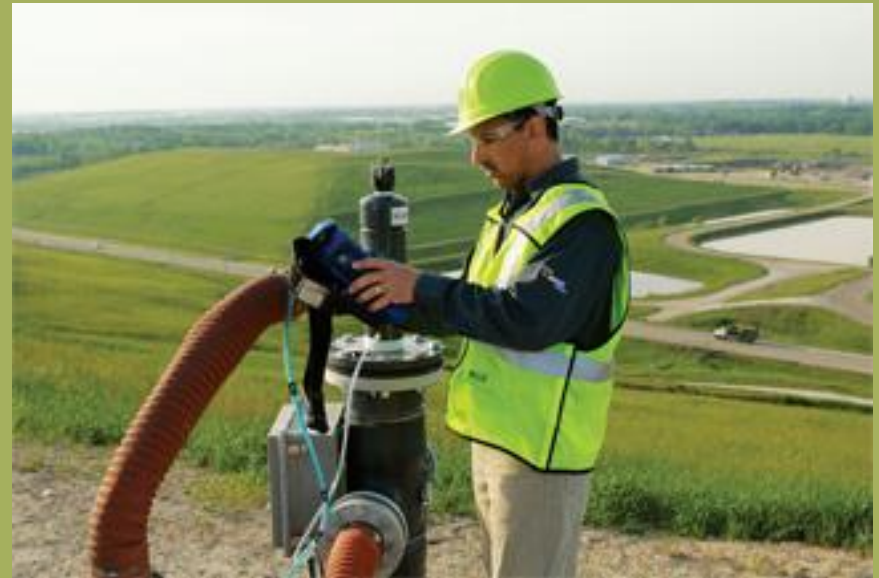
Landfill Gas Collection System
