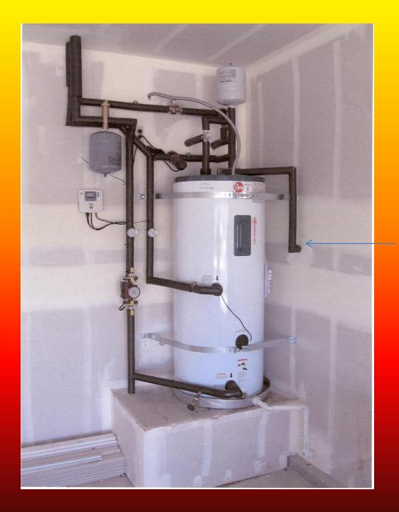
Pressure Relief Piped to Drain
