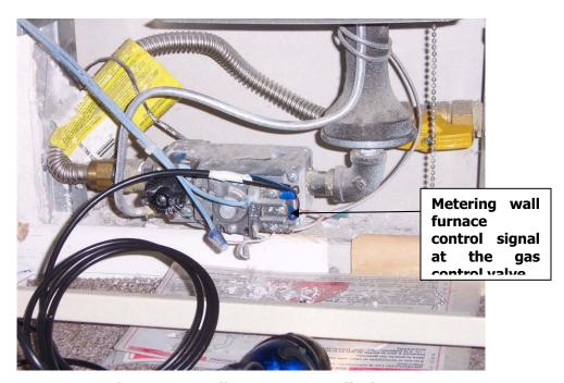
**Figure 66: Wall Furnace Installation**
