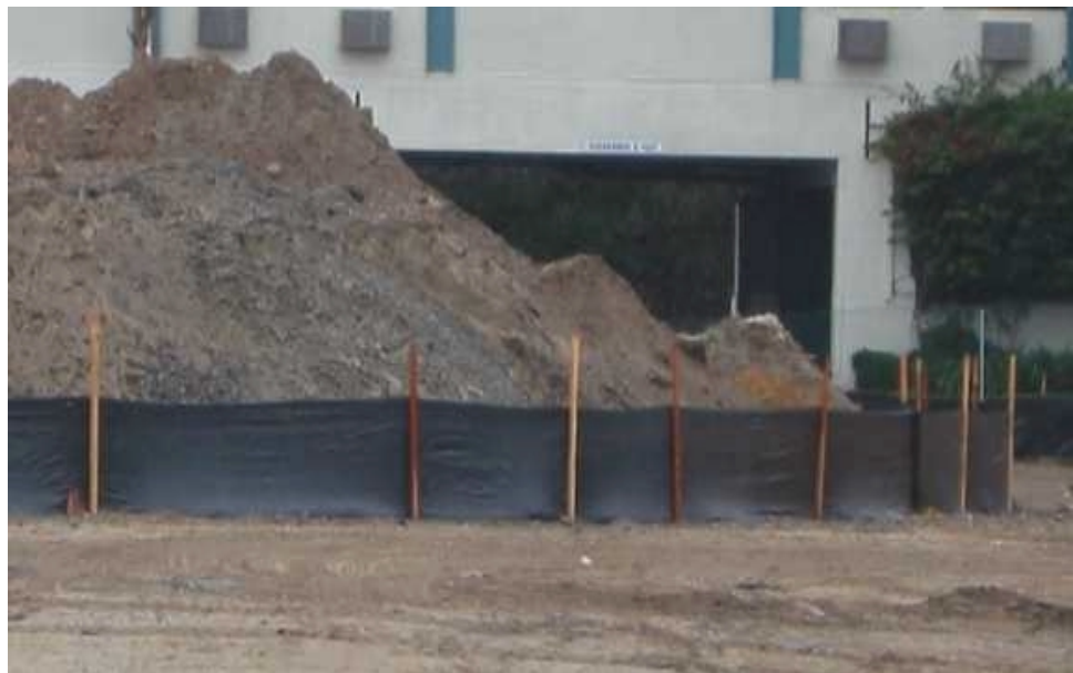
Silt fence used for stockpile perimeter control.
