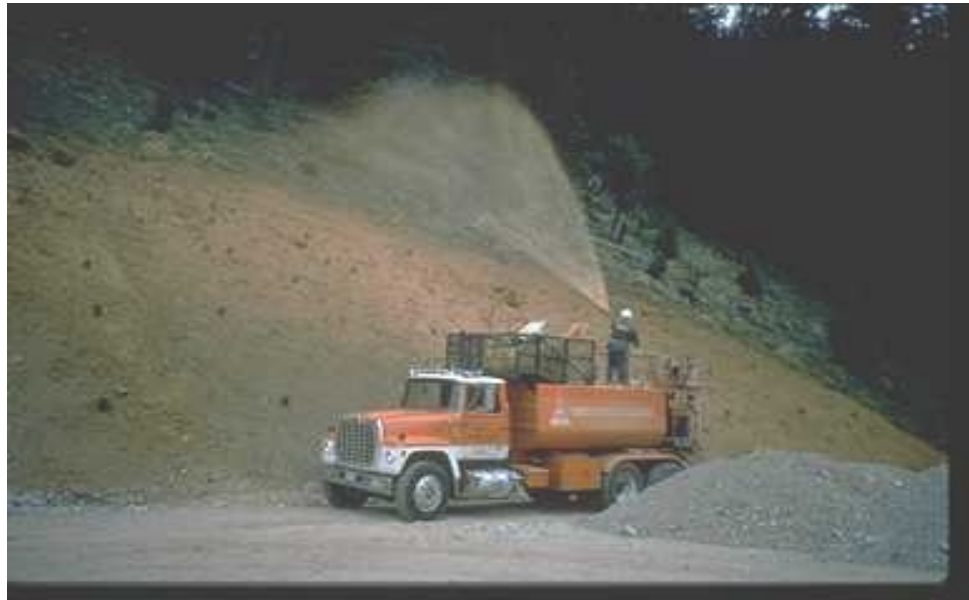
Applying hydraulic mulch.
