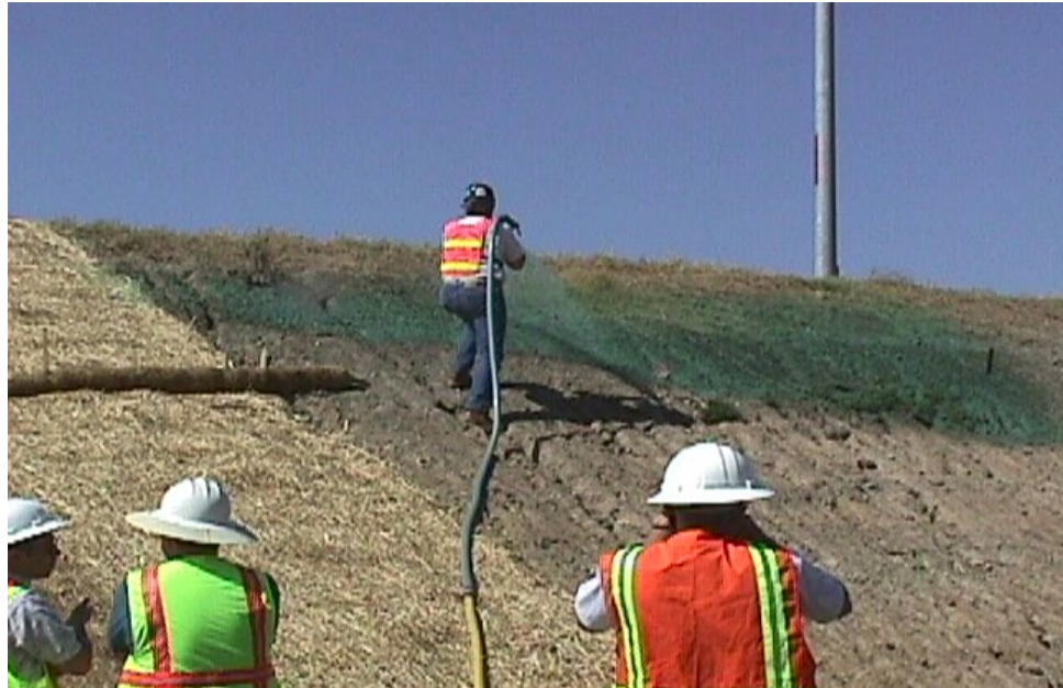
Applying soil stabilization manually in harder to reach areas.
