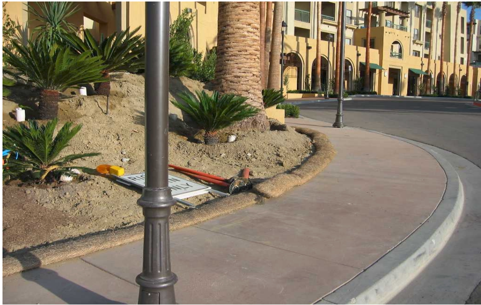
Fiber rolls as perimeter control
