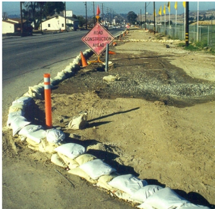
Sand bags used as perimeter control.
