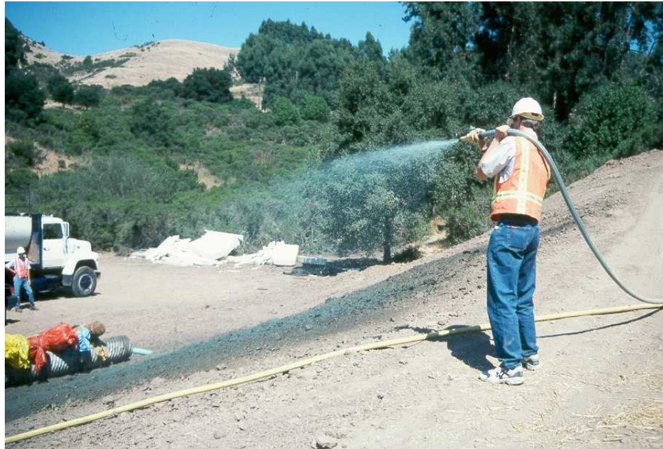
Applying hydroseed.
