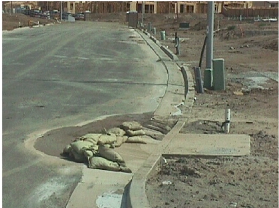
Gravel bag inlet protection.
