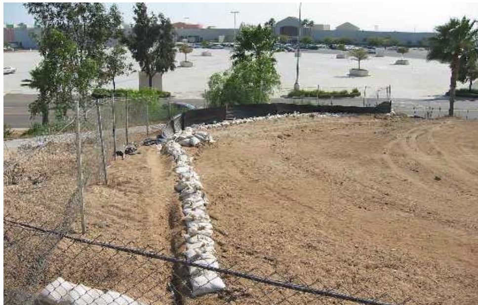
Gravel bags used as perimeter control.
