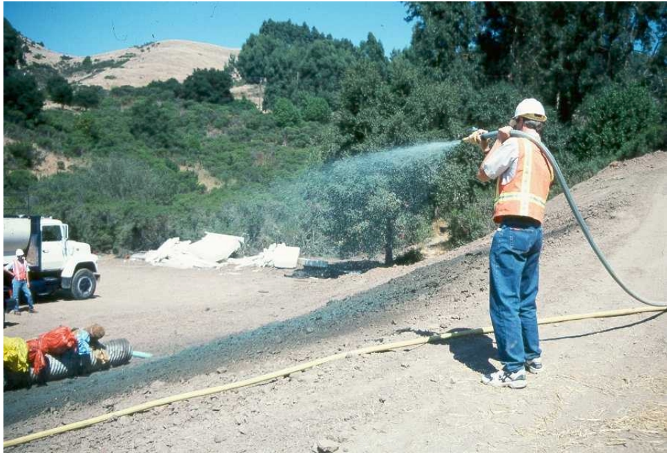
Applying hydroseed.
