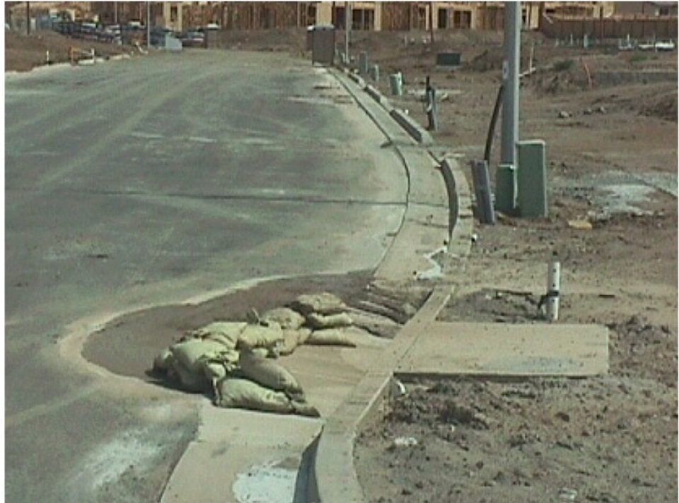
Gravel bag inlet protection.
