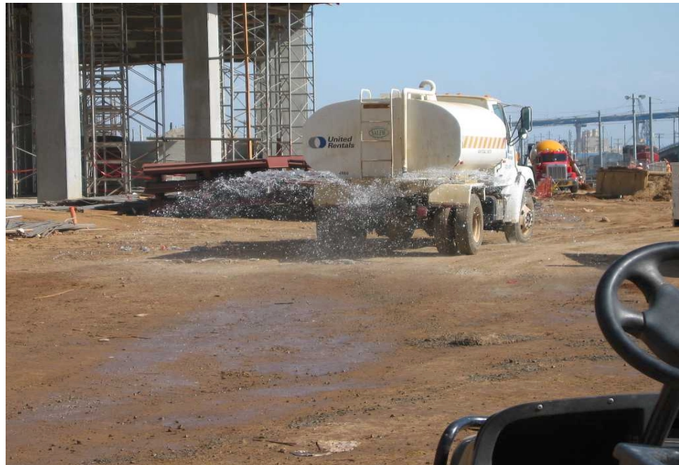
Water being applied for dust control.
