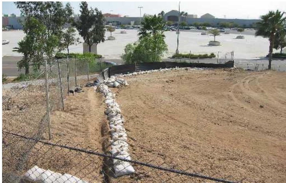
Gravel bags used as perimeter control.
