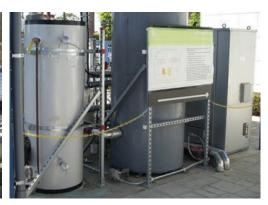
The solar thermal system at SoCalGas includes two types of concentrated solar collectors. One is a parabolic trough and the other uses Fresnel lenses and incorporates concentrated photovoltaics that produce electricity (cogeneration). The system also contains a hot water storage tank, an absorption chiller and a condensing hot water heater.
