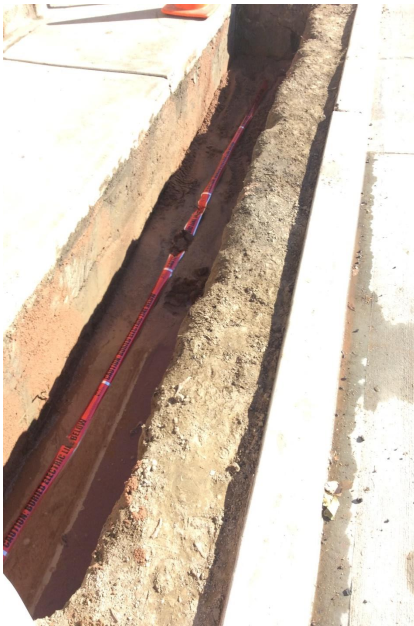
Figure 6: Lampson and Topaz – New Electrical Trench Prior to Backfill
