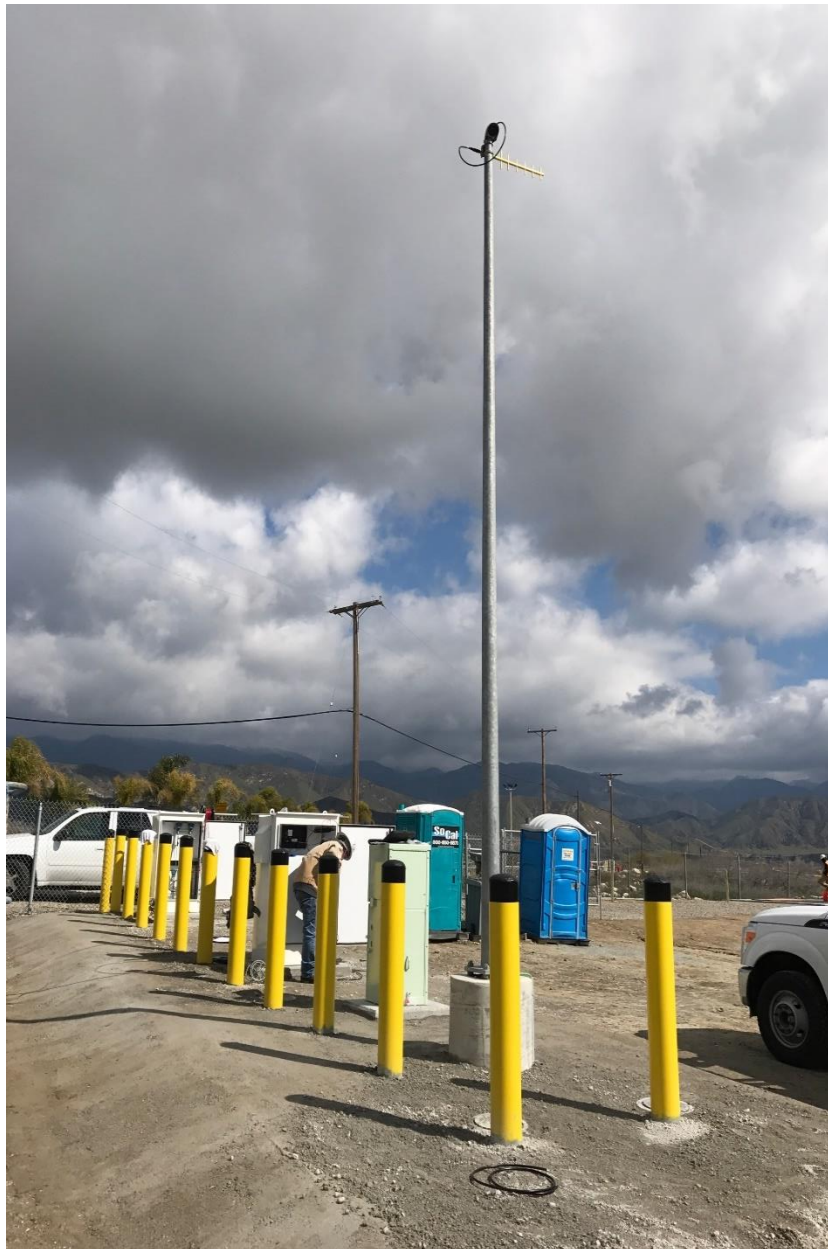
Figure 3: New Communications Antenna
