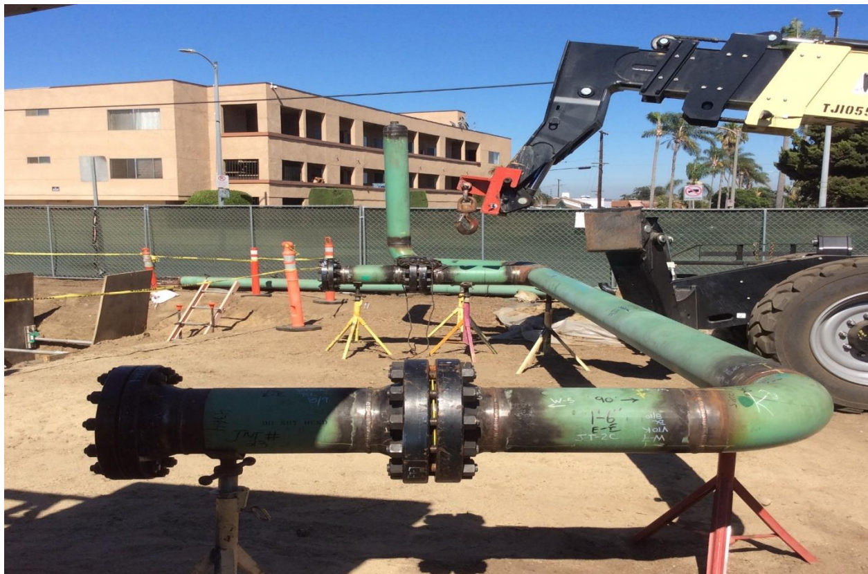
Figure 7: Vermont Avenue and 102 nd Street – New Blowdown Assembly Prior to Installation
