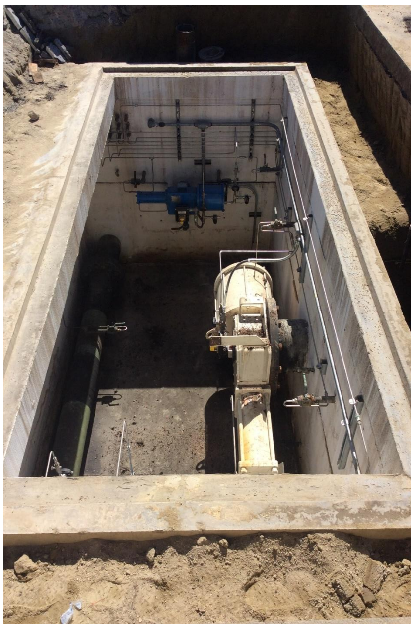
Figure 5: Lampson and Pine – New Vault and Actuators
