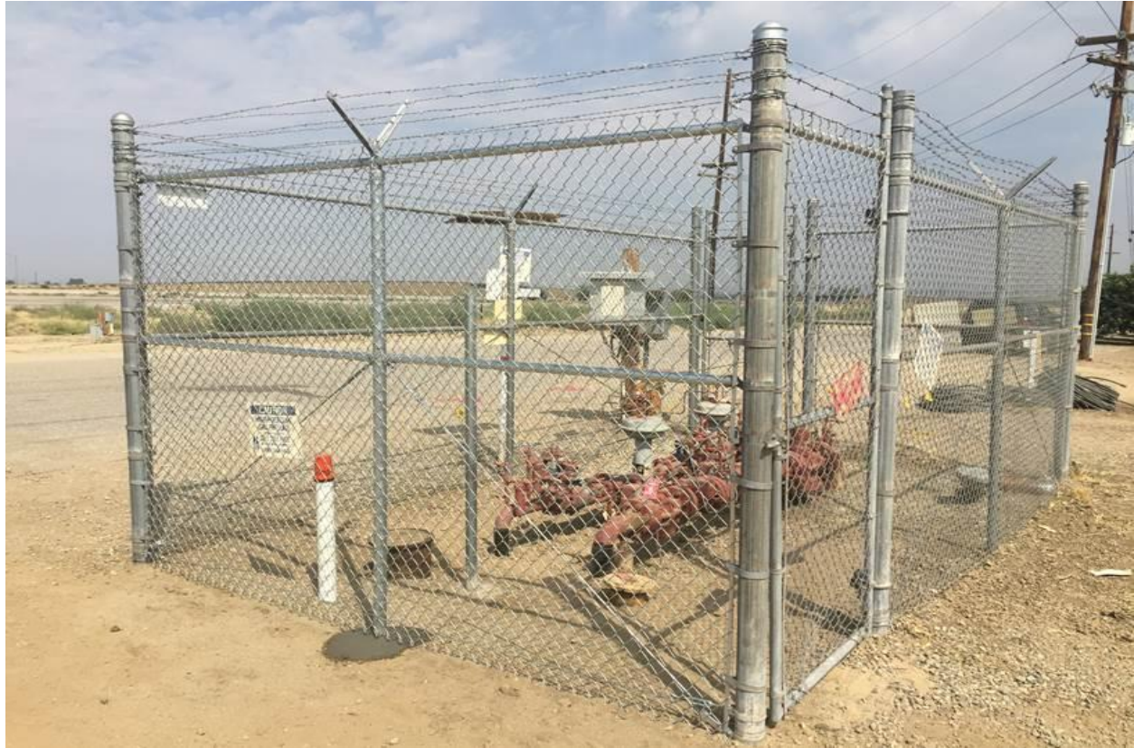
Figure 6: A Street – Post Construction
