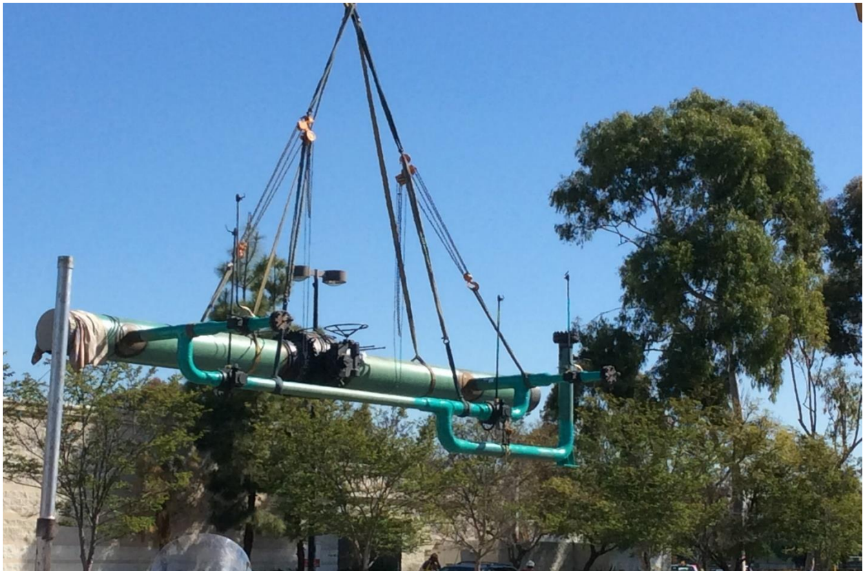
Figure 6: Bloomfield Avenue Project Site – New Mainline Valve and Blowdown Assembly Installation
