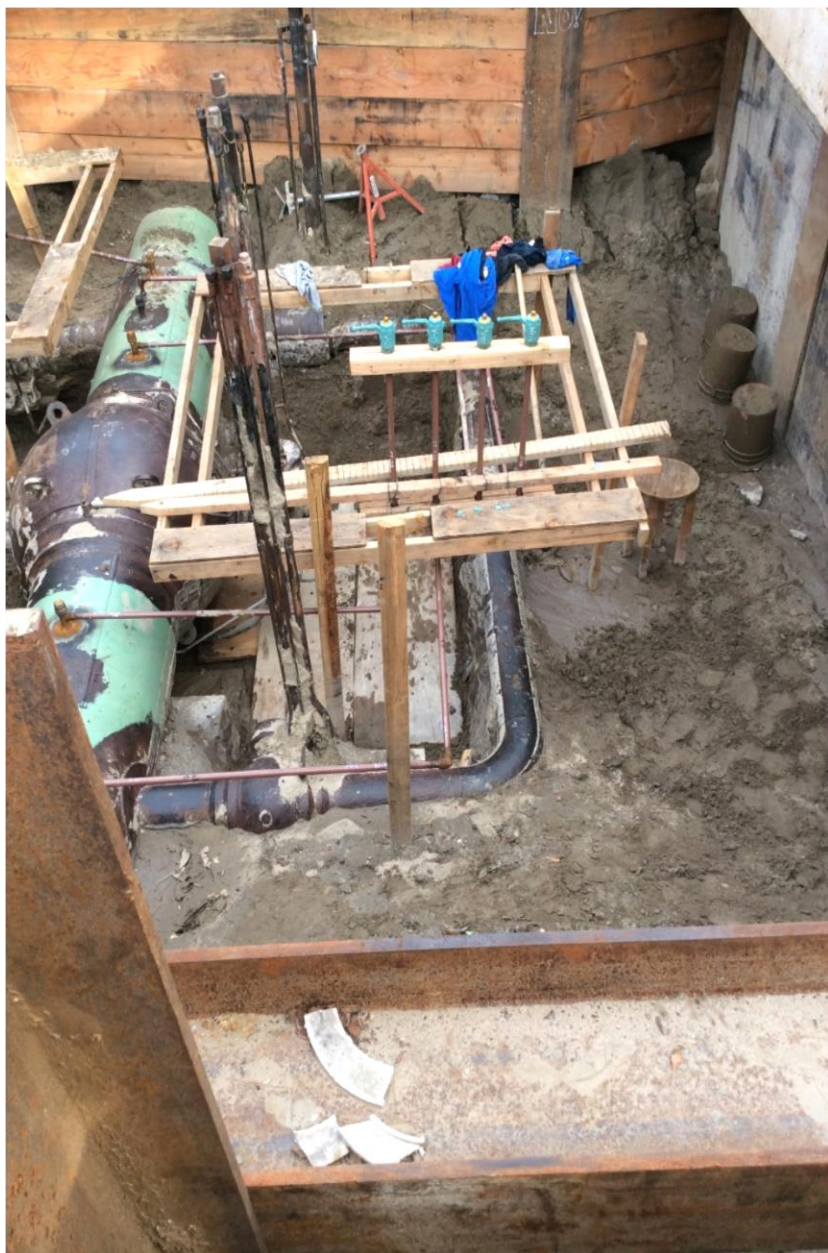
Figure 5: Brookhurst Street Project Site – Mainline Valve Excavation
