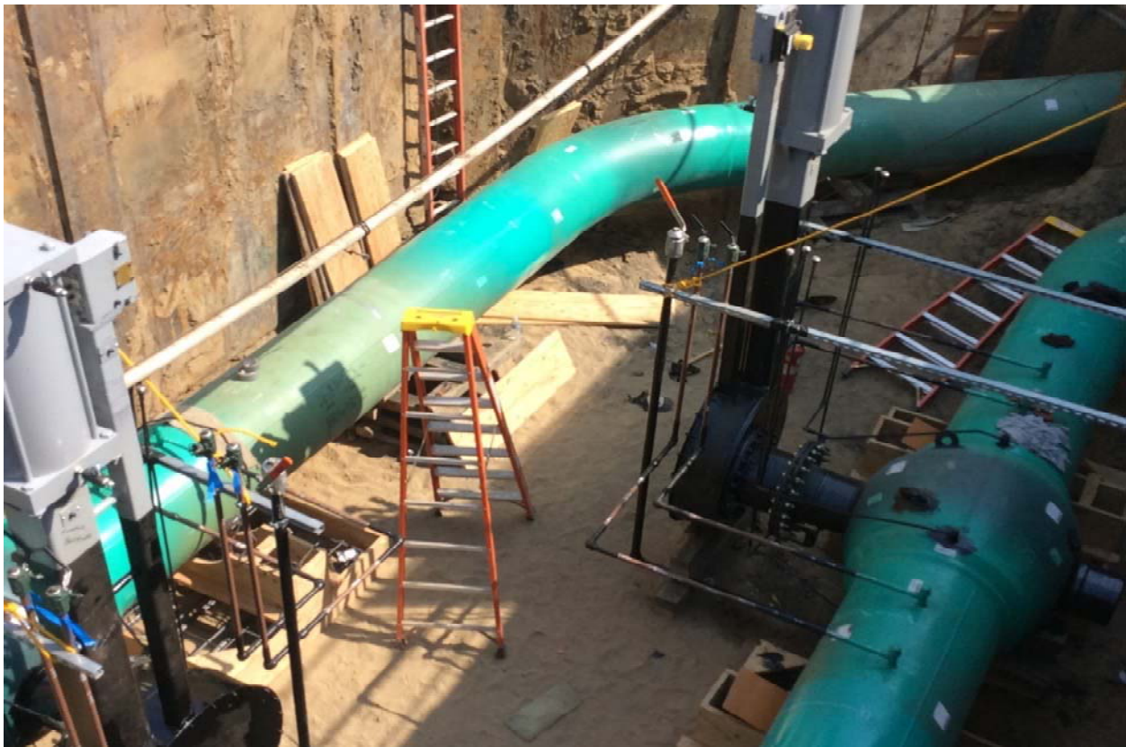
Figure 3: New Mainline Valves After the Tie-in with New Actuators
