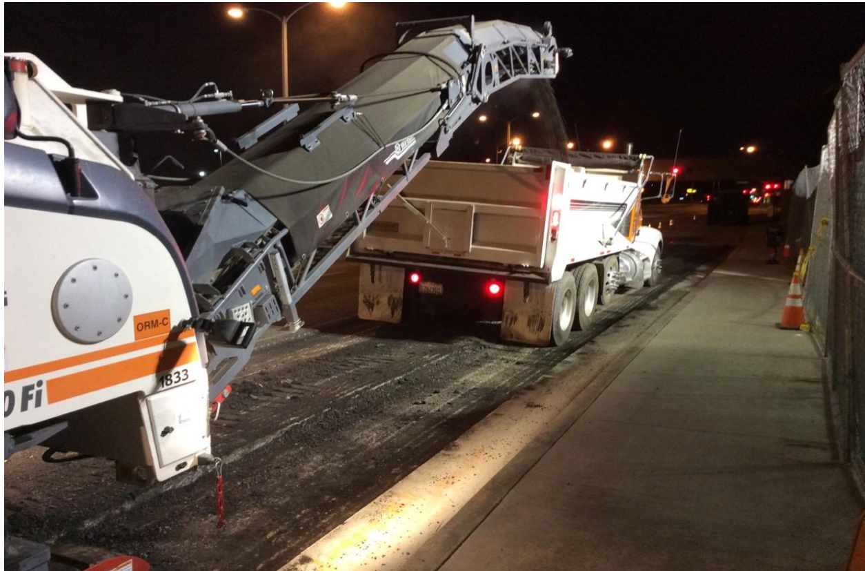
Figure 5: Nighttime Resurfacing of El Segundo Boulevard
