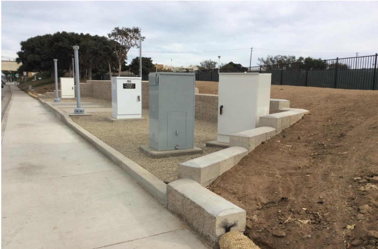
Figure 4: New Cabinets, Vaults, Retaining Wall, and Sidewalk
