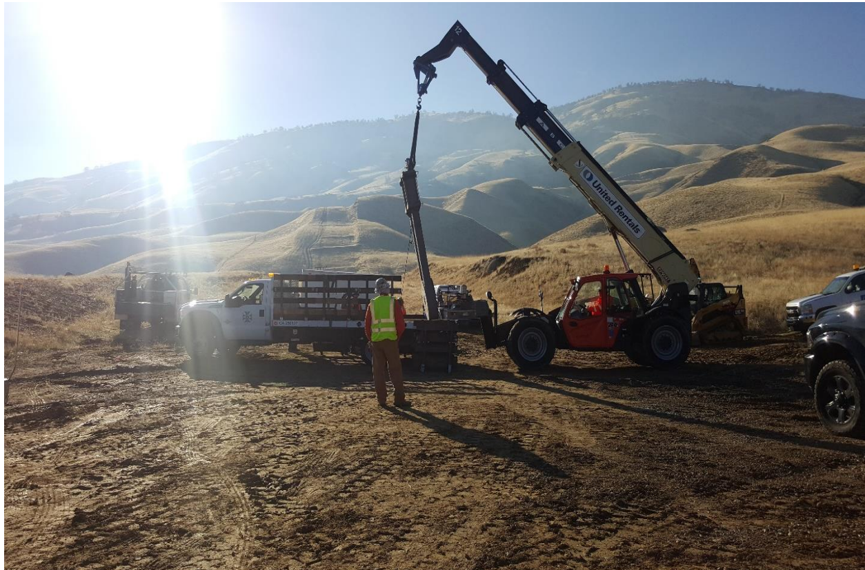
Figure 8: Line 225 Valve Enhancement Project Bundle – Edmonston: Unloading of the New Actuator
