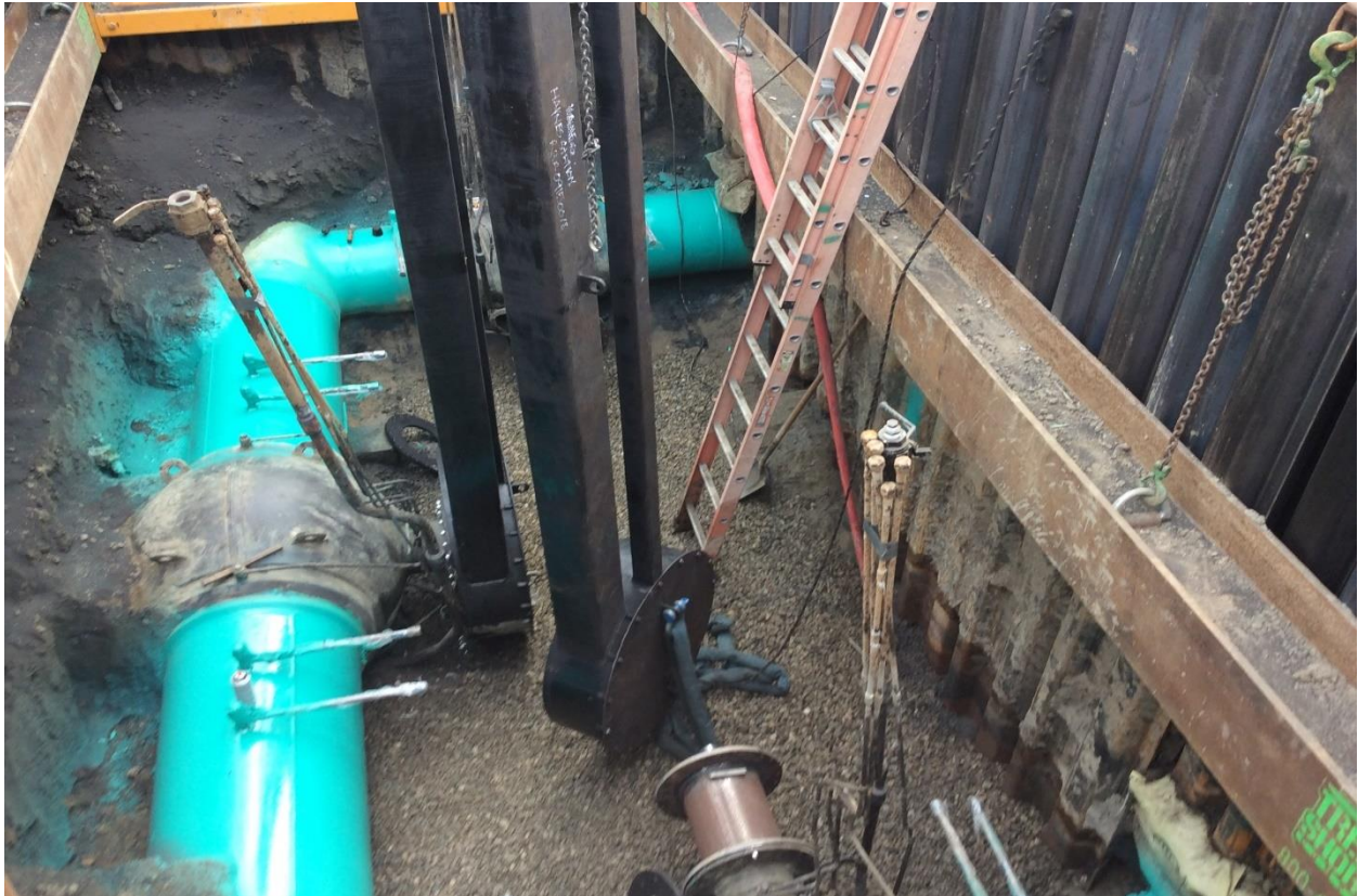
Figure 3: Mainline Valve Excavation and New Actuator
