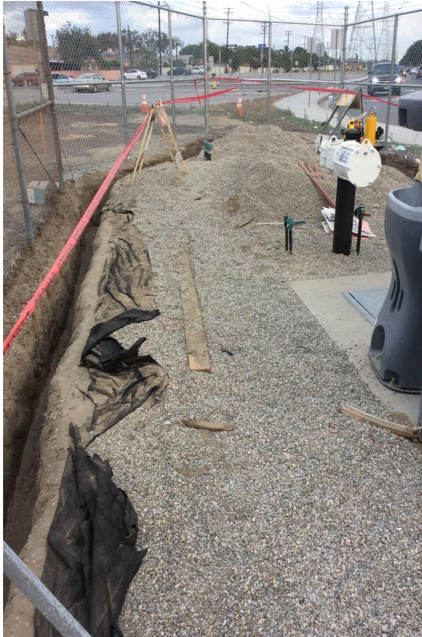
Figure 8: Southern and Alameda – New Actuator and Trenching for Station Grounding Installation
