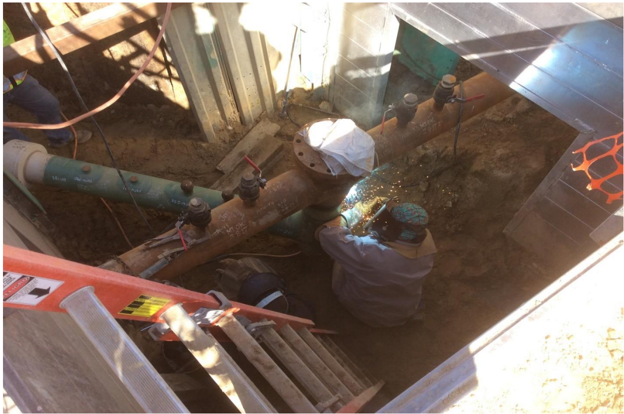
Figure 5: Tie-In to Existing [REDACTED] Line
