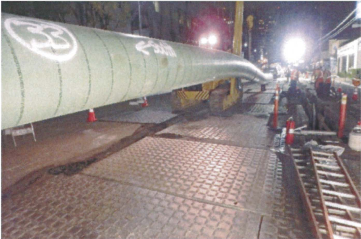
Figure 7: Preparing Pipe String for Installation in Trench
