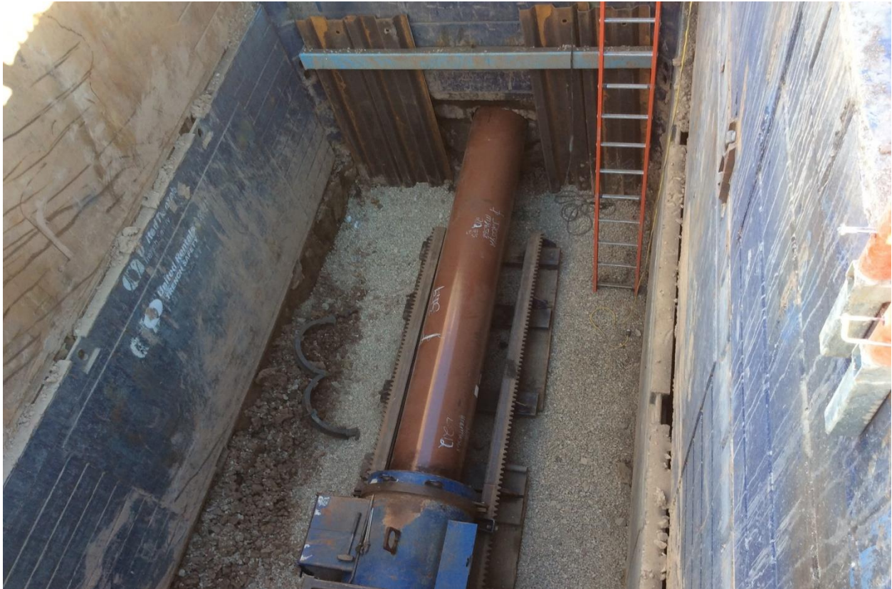
Figure 6: Boring Machine Pushing ██████████ Abrasive Resistance Overcoat Pipe
