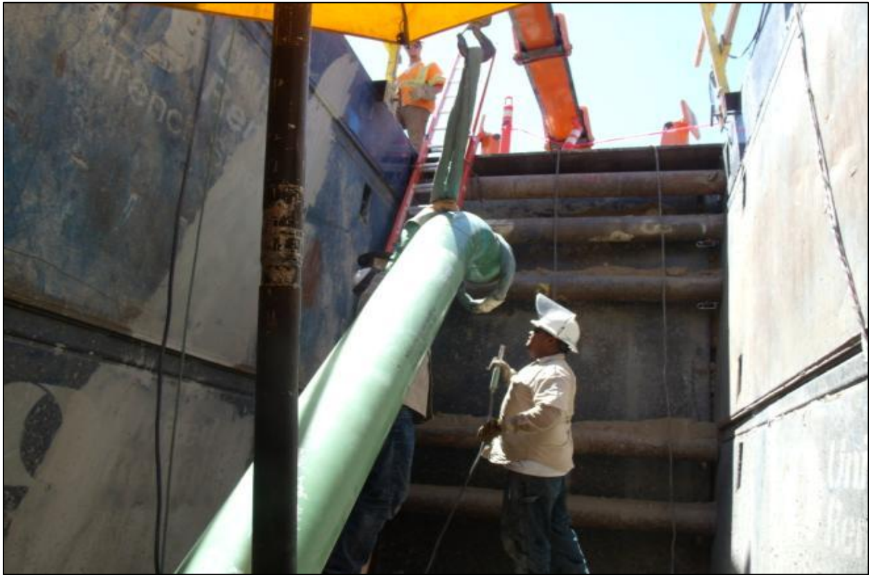
Figure 7: Section 2 - Bore Pit
