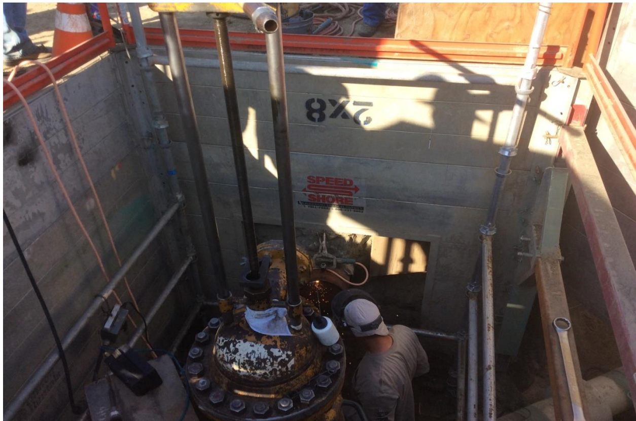
Figure 7: Welding Plate on Abandoned [REDACTED] Line
