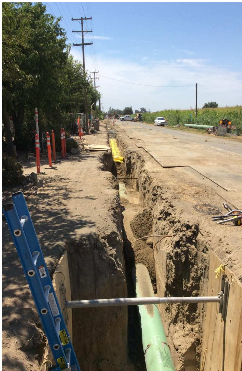
Figure 11: Backfilling the Pipeline Trench
