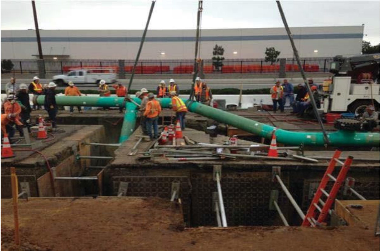
Figure 9: Lowering Section of Pipe into Trench
