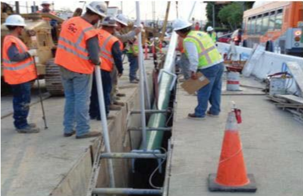
Figure2: Lowering Pipe in Congested City Area
