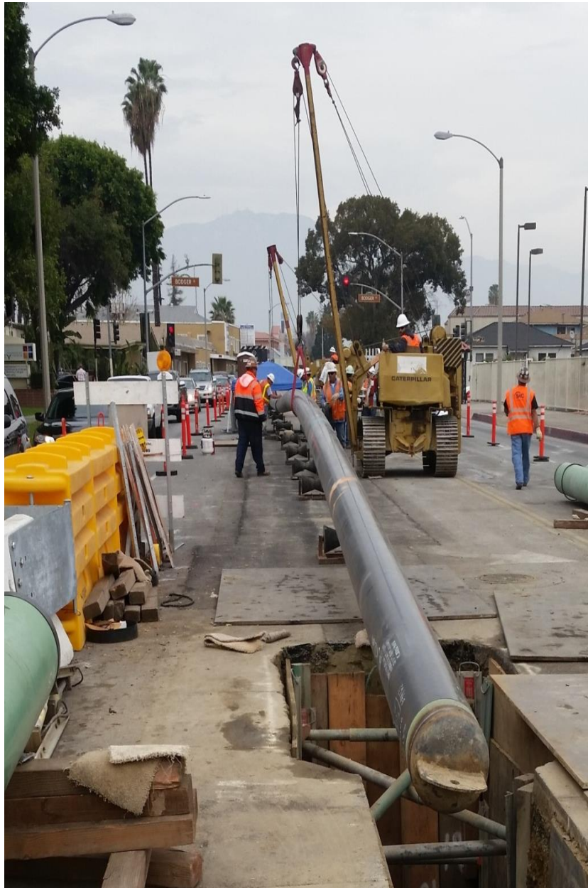
Figure 3: Shallow HDD Pullback Preparation at Santa Anita Avenue and MTA Way
