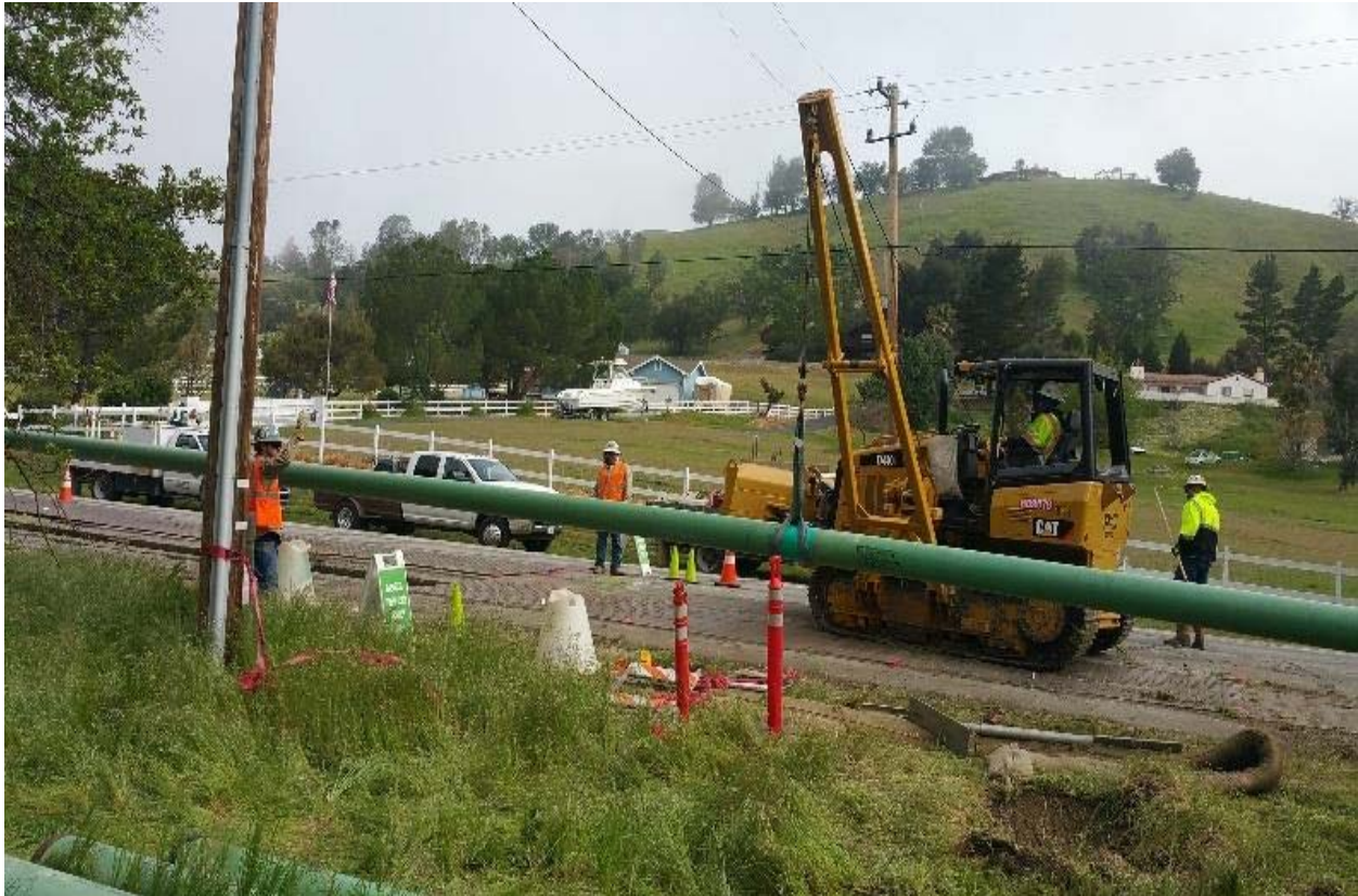
Figure 4: Spotter Signaling to Operator Overhead Wires
