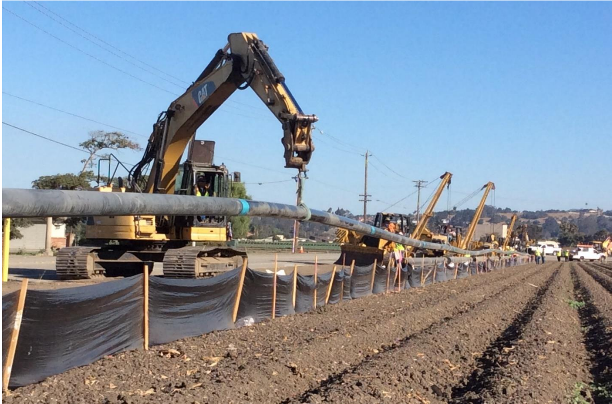
Figure 13: Section 7A - HDD Pipe Lifted for Transport to HDD Entry Point
