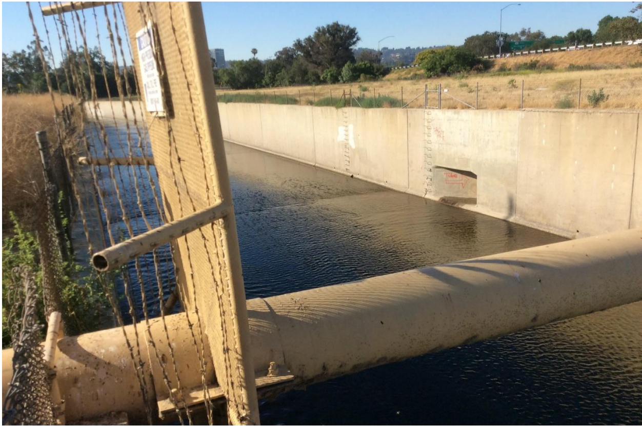
Figure 3: Span Crossing of Abandoned Bypass
