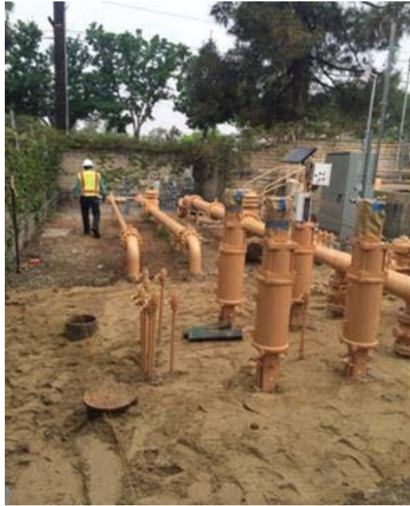
Figure 18: Large Valve Station with Numerous Above-Ground Features
