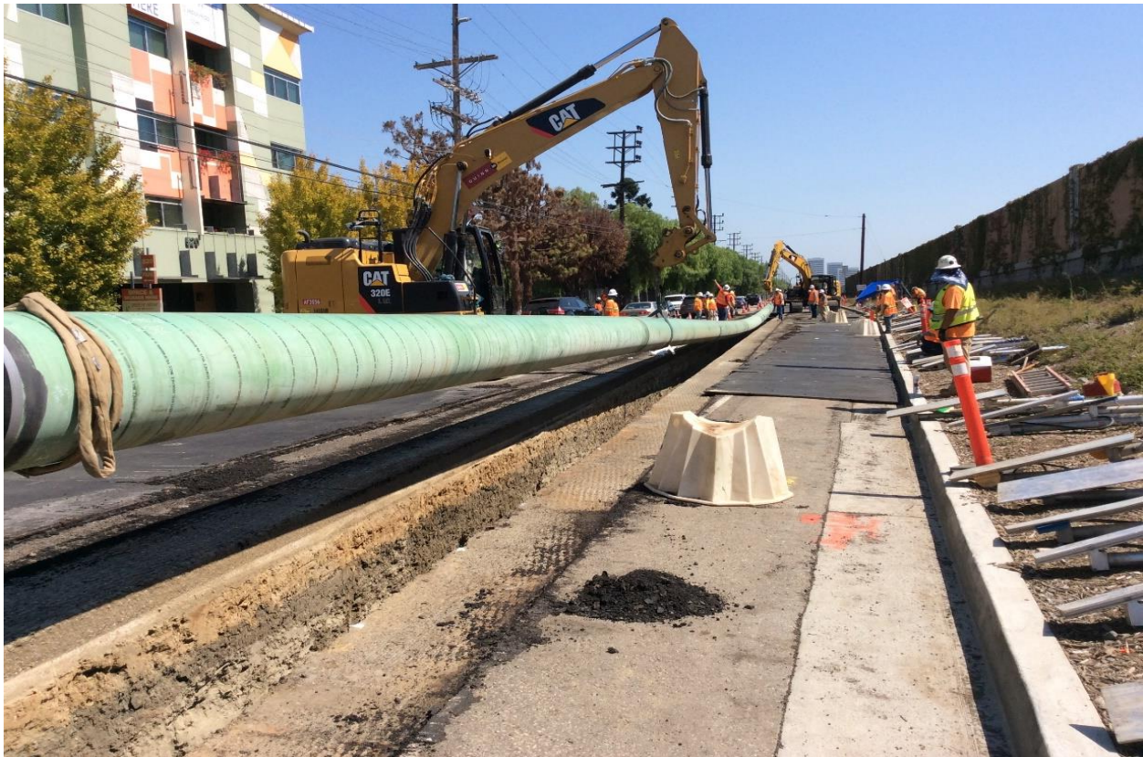
Figure 5: Installing Pipe String into Trench
