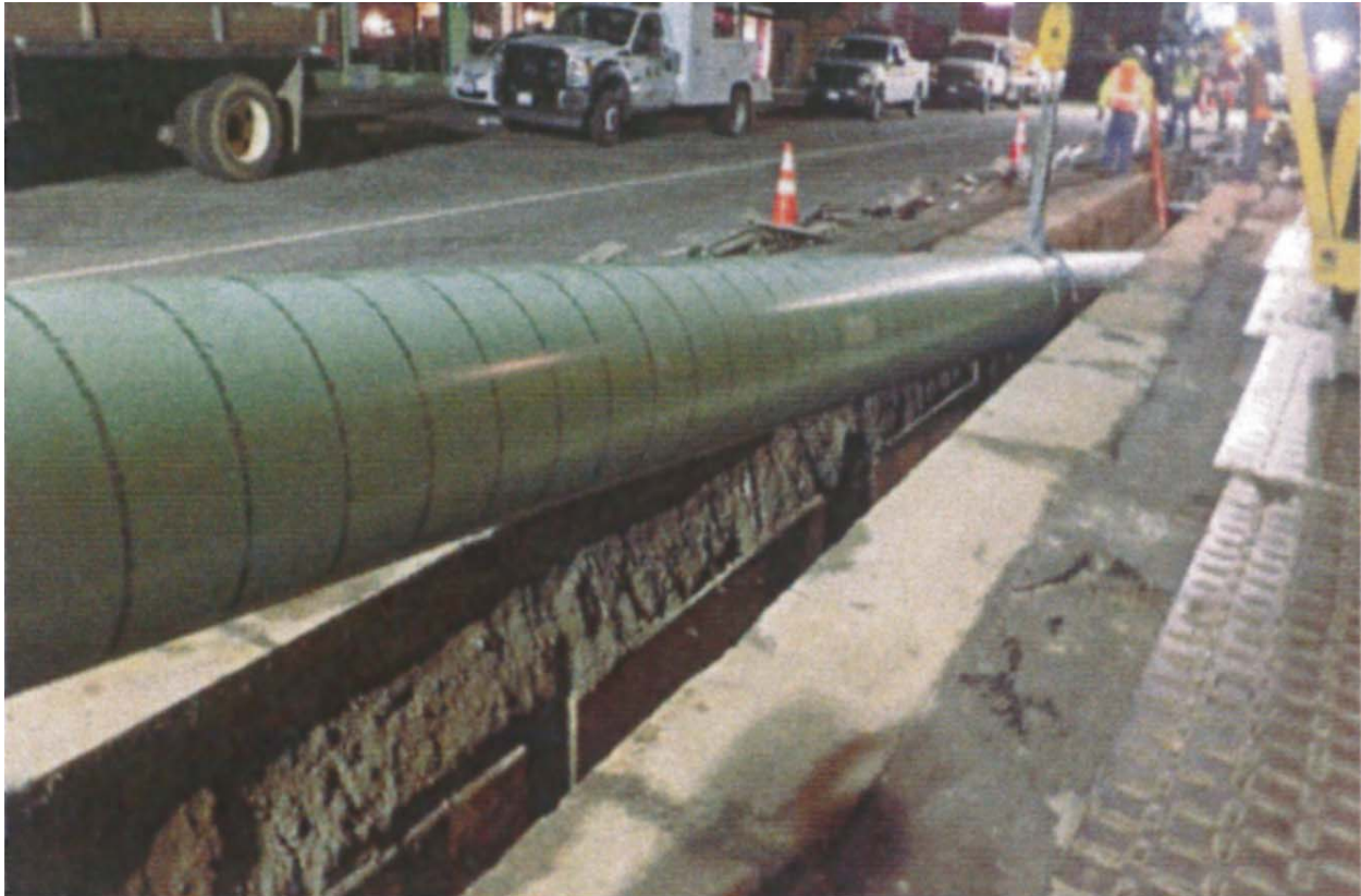
Figure 8: Laying Pipe String in Trench
