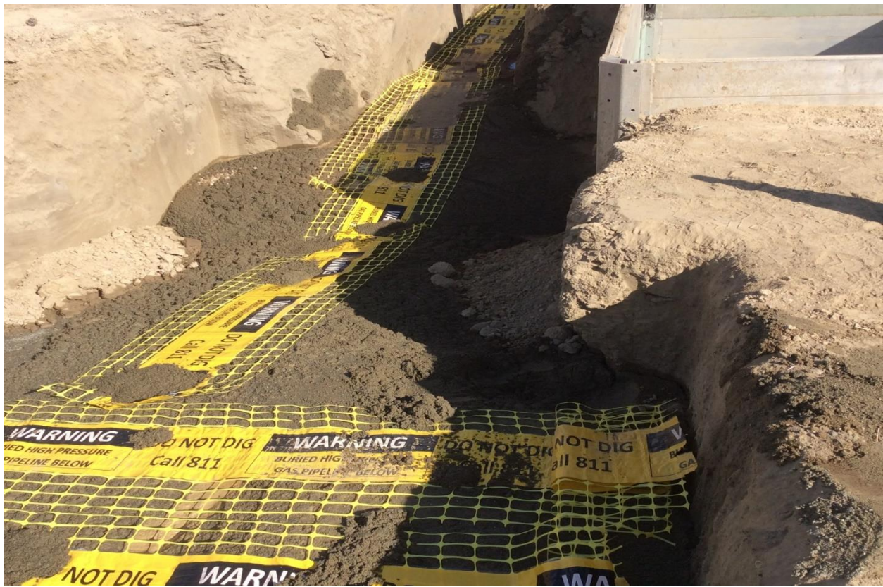
Figure 5: Backfill and Warning Mesh
