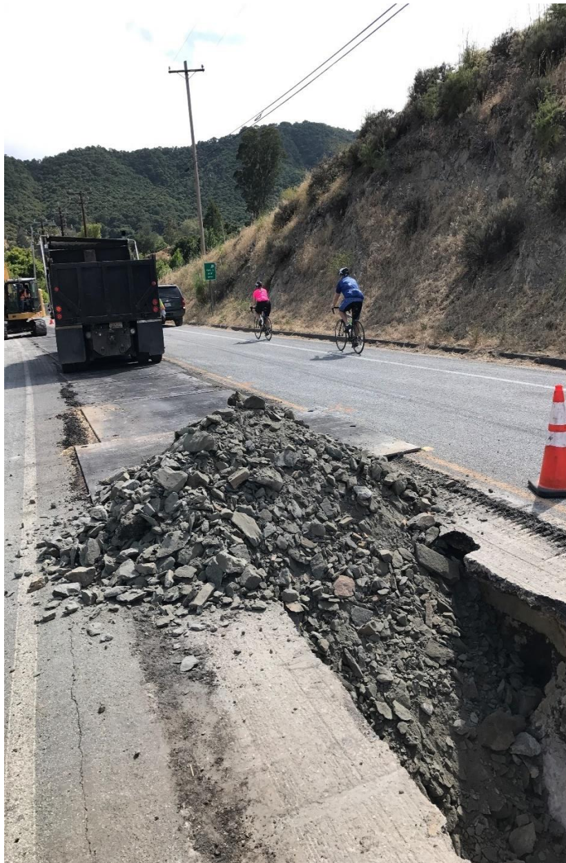
Figure 10: Broken Rock for New Pipe Installation
