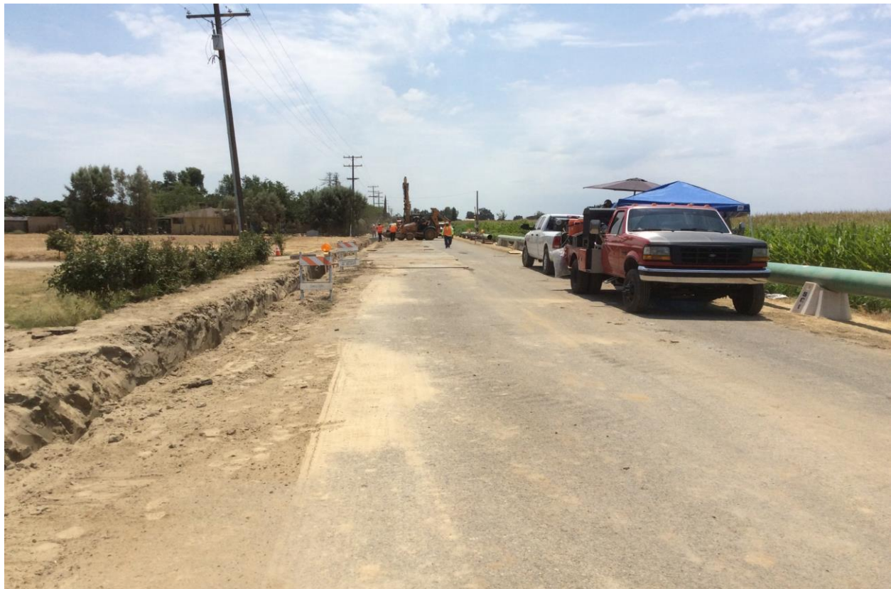
Figure 10: Elm Avenue During Construction
