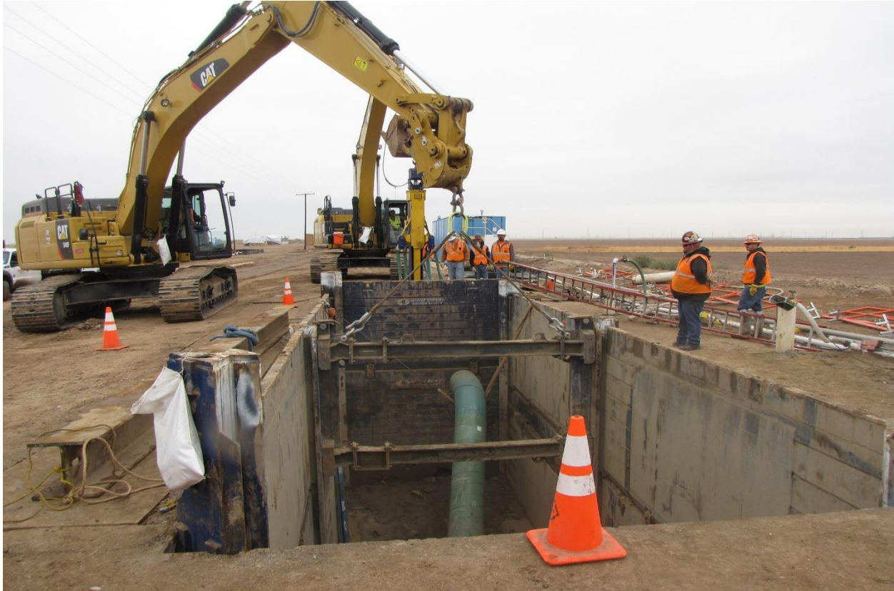
Figure 7: Pipe Tie-in Complete and Preparation of Bore Pit for Backfill
