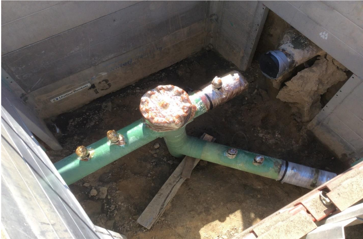
Figure 9: Fittings Wrapped
