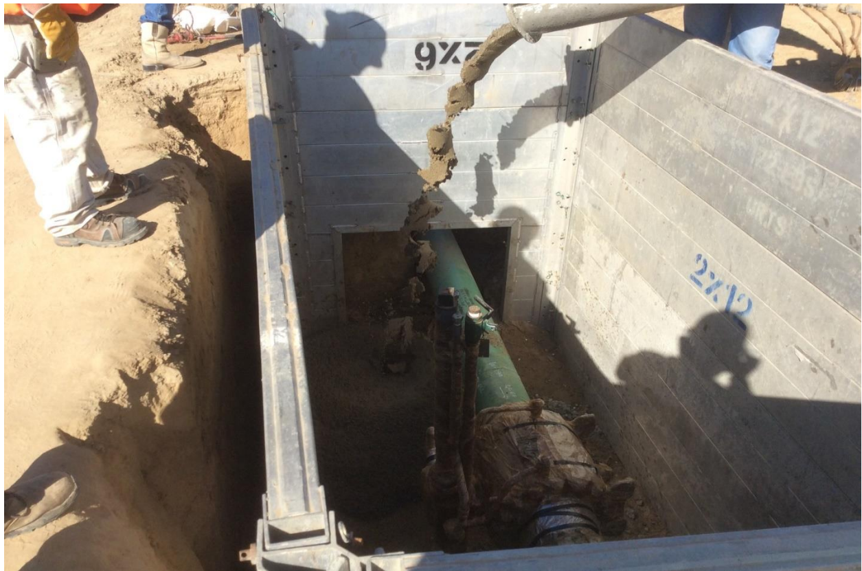
Figure 10: Slurry Backfill
