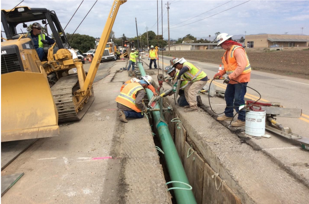
Figure 14: Section 7A - Lowering Pipe into a Trench
