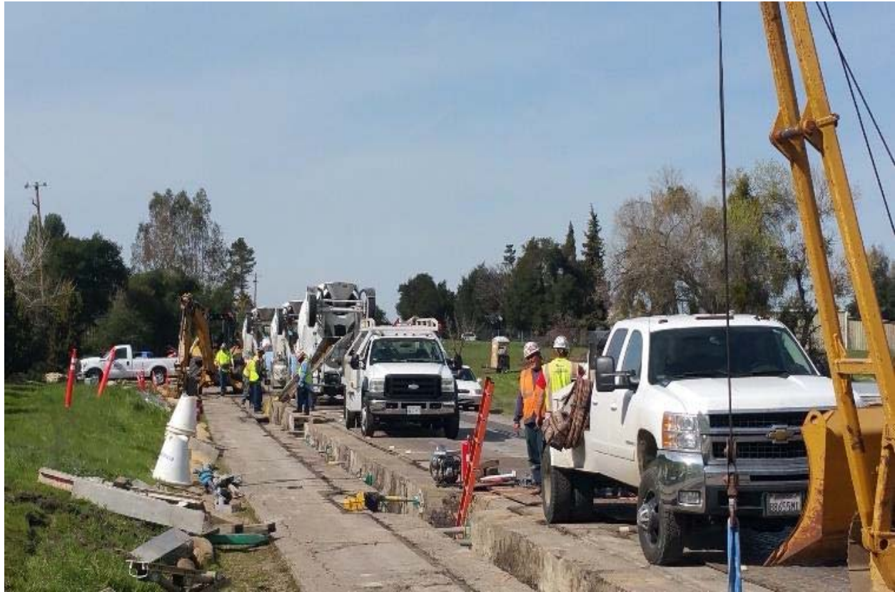
Figure 5: Slurrying New Pipeline
