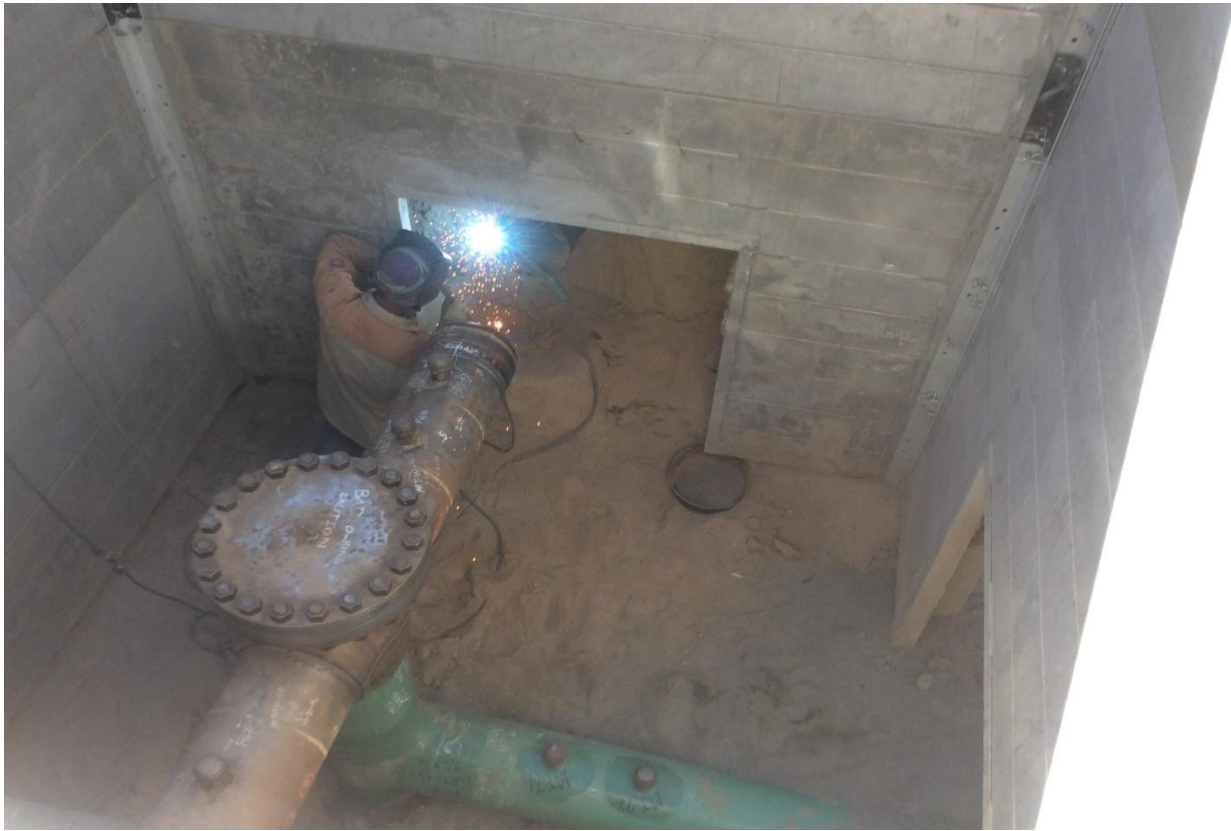
Figure 4: Closure Plate Installation on Abandoned [REDACTED] Supply Line
