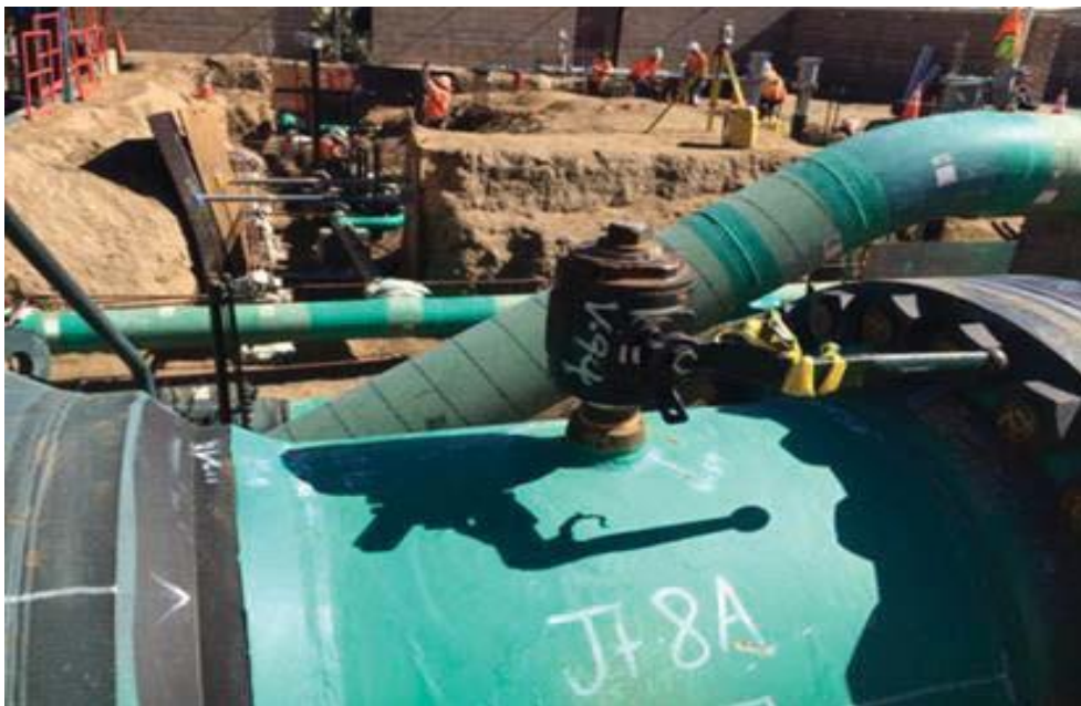
Figure 18: Large Valve Station with Numerous Above-Ground Features
