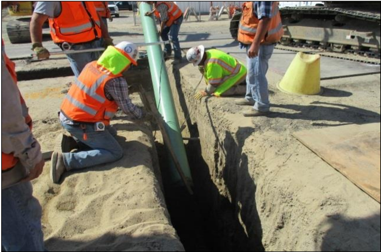
Figure 9: Section 2 - Lowering Fabricated Section of Pipe into Trench with Sugar Sand
