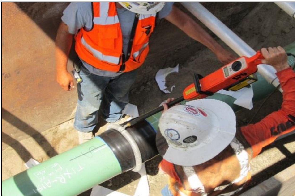
Figure 8: Section 2 – Checking Integrity of Coating
