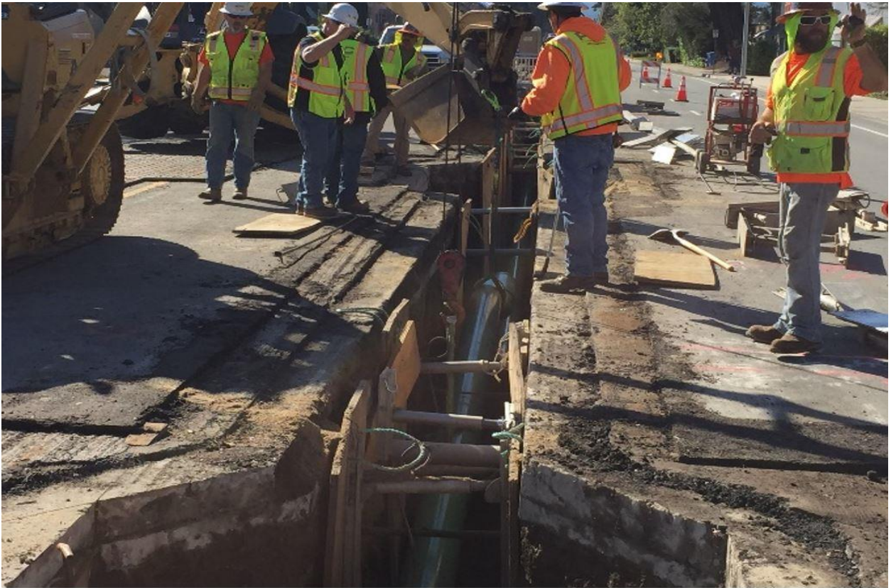
Figure 4: Installation of Pipe along South Higuera Street
