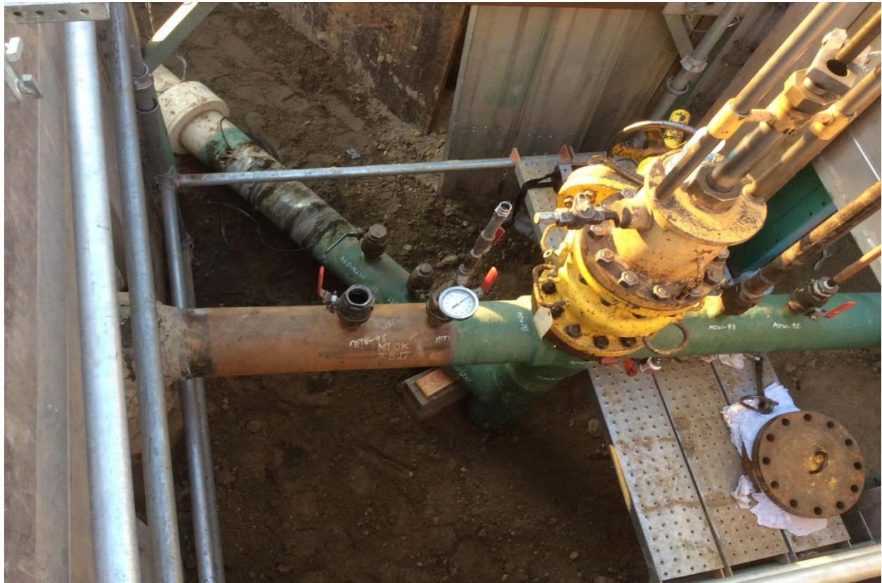
Figure 8: [REDACTED] Line Prior to Cut and Cap
