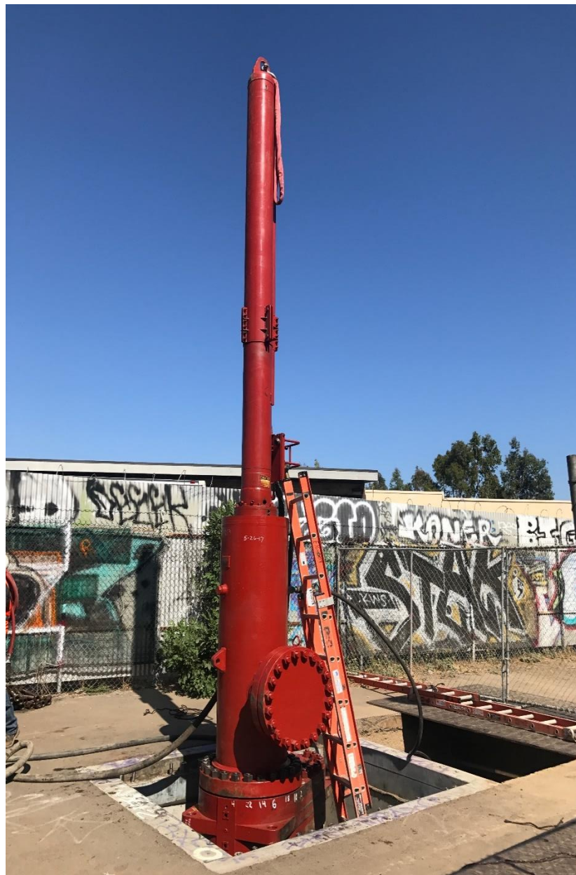
Figure 6: Pressure Control Fitting Isolation Machine
