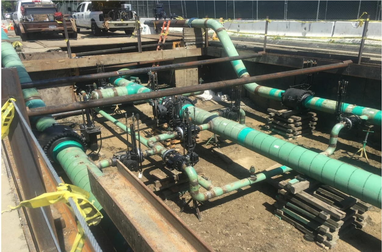
Figure 7: Replacement Bridle Configuration During Construction
