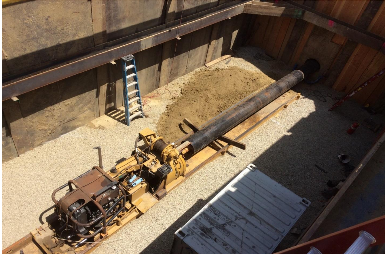
Figure 6: Jack-and-Bore Construction Set Up
