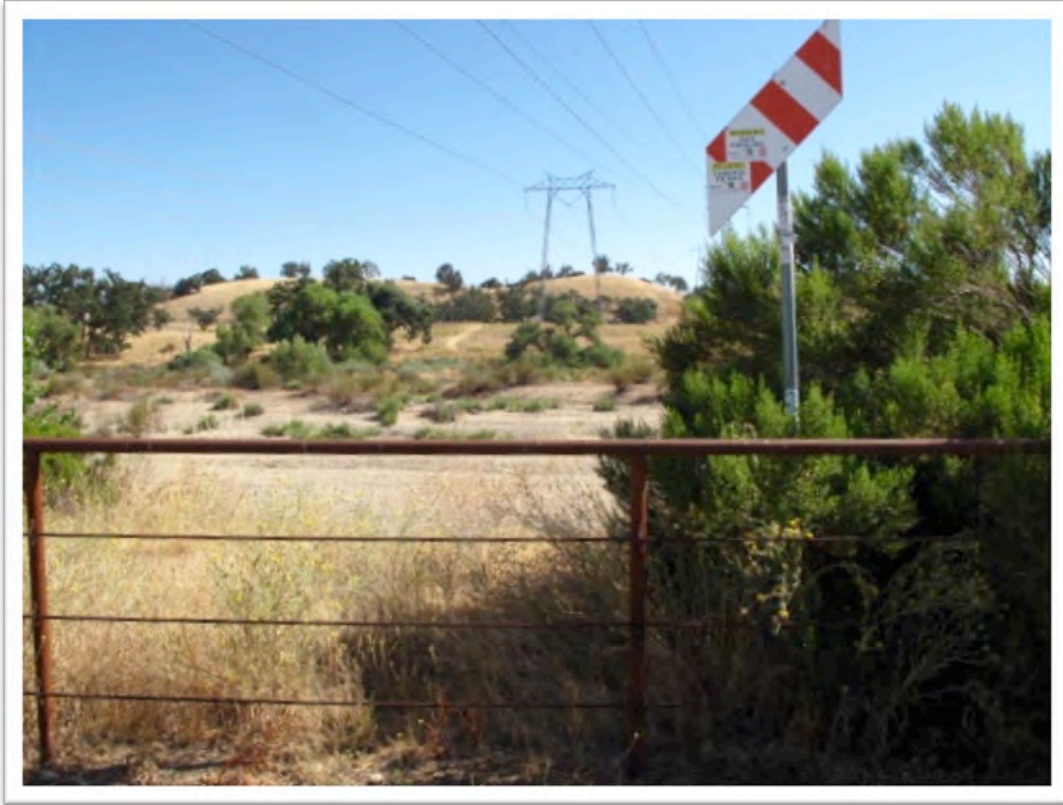
Figure 28. Dry Creek crossing south of Paso Robles on right-of-way looking north.
