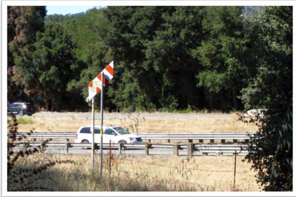
Figure 30. Line 306 crossing at Highway 101 looking south near Paso Robles.
