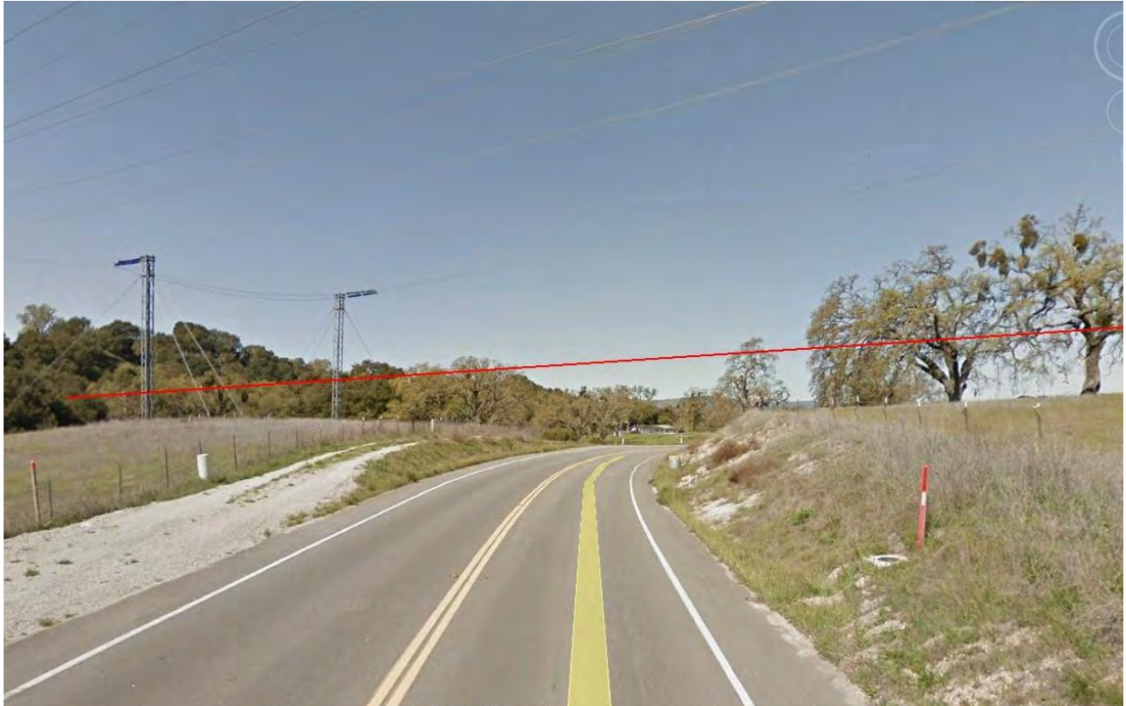
Figure 13 – Morro Bay ■ Gas Pipeline System – Crossing Templeton Rd
