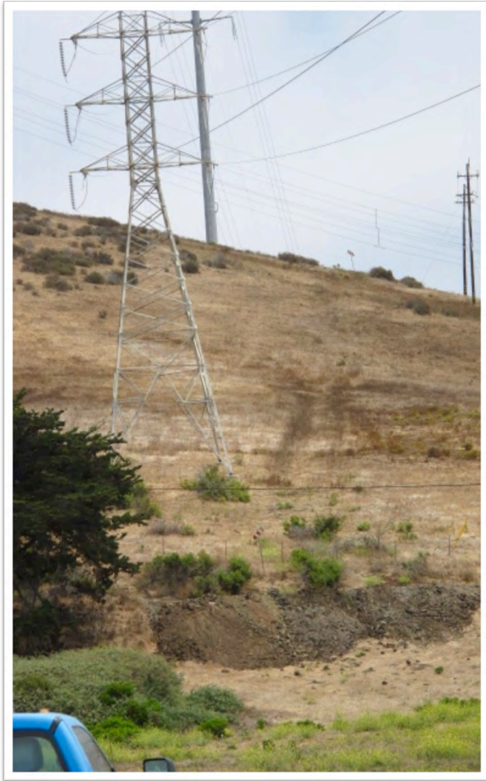
Figure 38. Right-of-way coming into Morro Bay Station.
