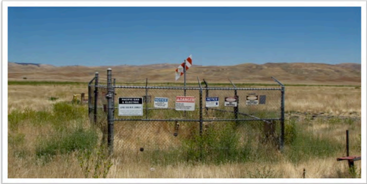
Figure 18. Hartfield Valve Station, the nearest facility to the San Andreas Fault line at milepost 26. This station is located on a plain between two hill ranges. This view of the station is looking eastward.
