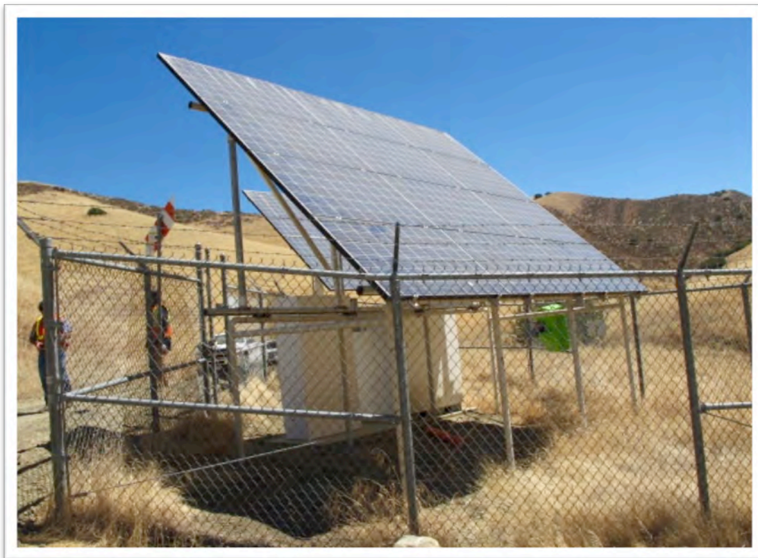
Figure 15. Solar powered rectifier station for Line 306 at [REDACTED]
