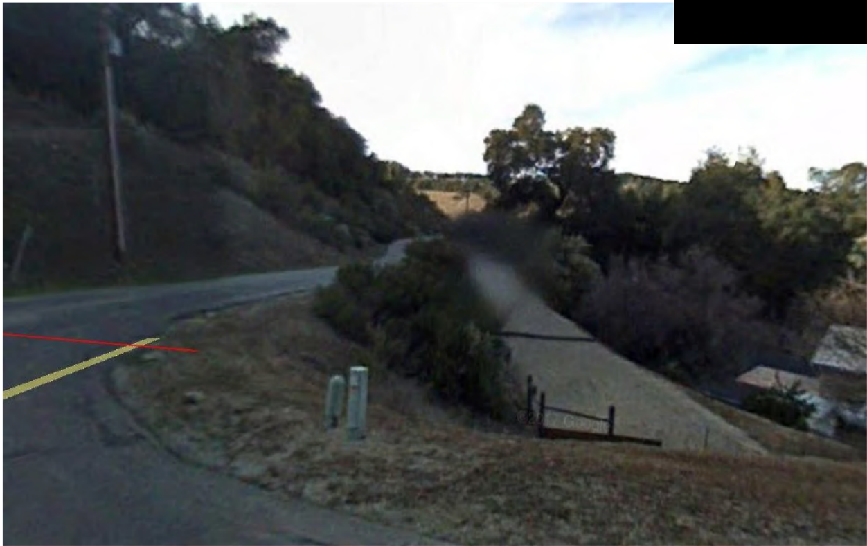
Figure 7 – Morro Bay [REDACTED] Gas Pipeline System – Crossing San Gregorio Rd
