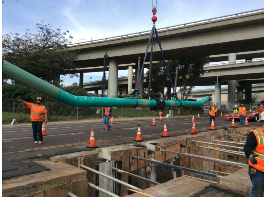
Figure 1: Construction Area in HCA
