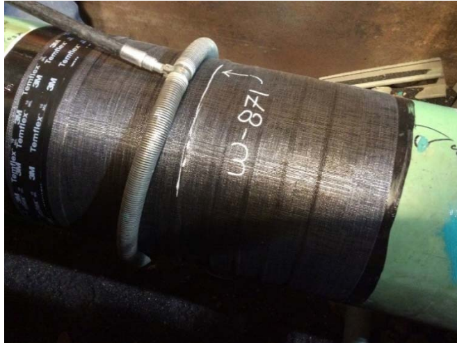
Figure 16: Holiday Testing of a Coated Weld
