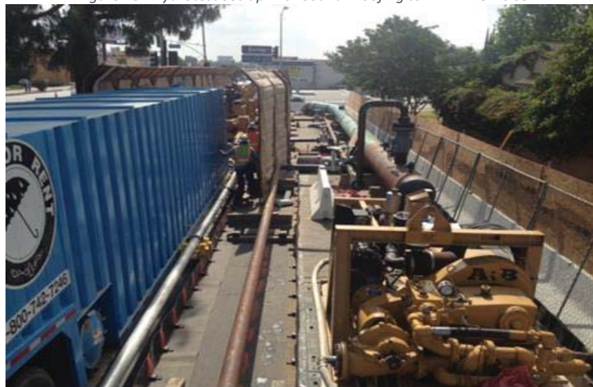
Figure 18: Hydrotest Set-up with Sound Proofing to Minimize Noise
