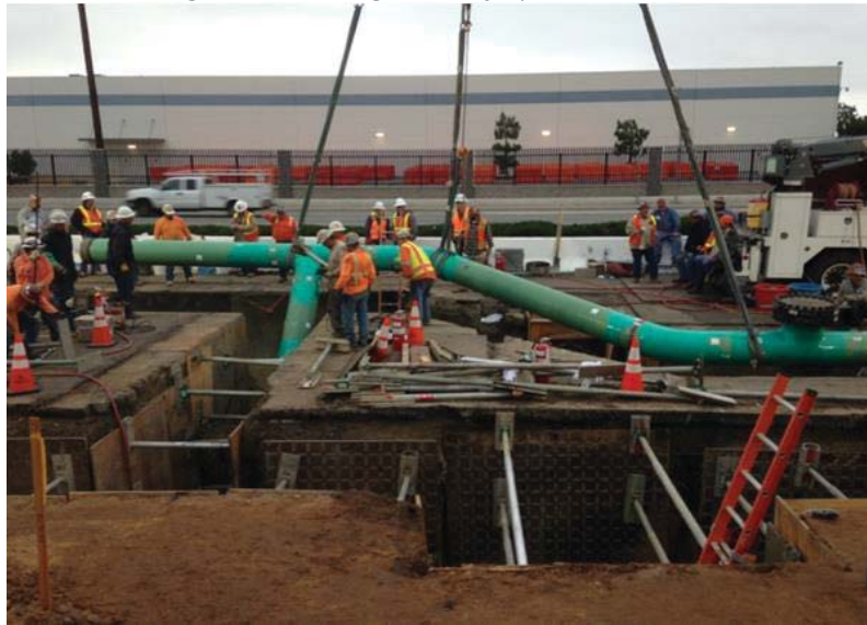
Figure 14: Lowering Section of Pipe into the Trench
