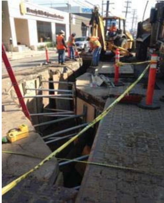
Figure 8: Shoring in an Urban Location
