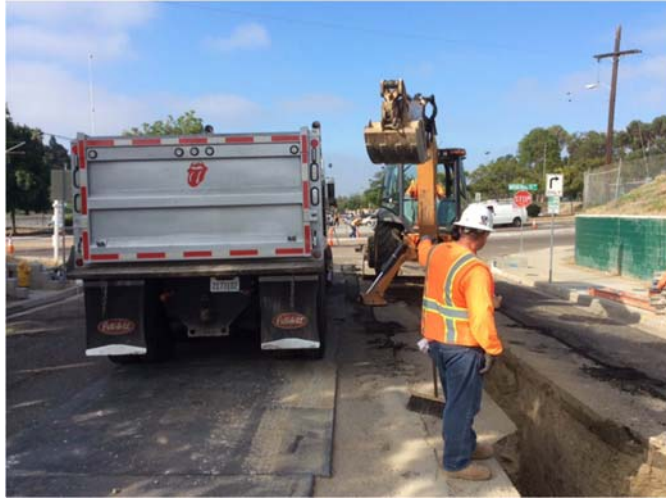
Figure 6: Excavation with Backhoe
