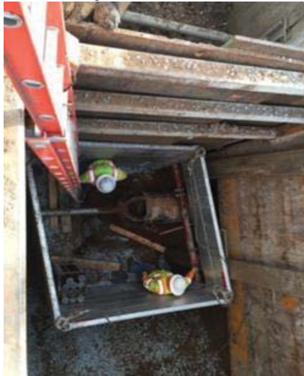
Figure 11: Jack and Bore Pit
