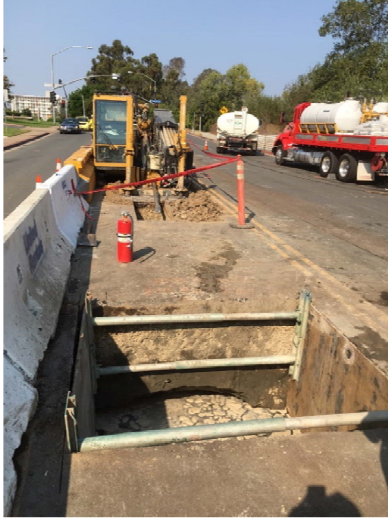
Figure 10: Highway 163 Horizontal Directional Drill (HDD) Crossing
