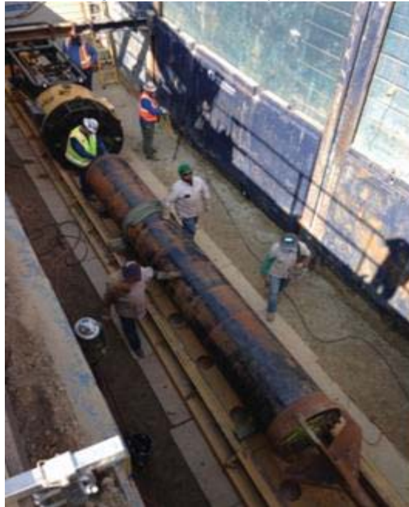
Figure 12: Jack and Bore Operations
