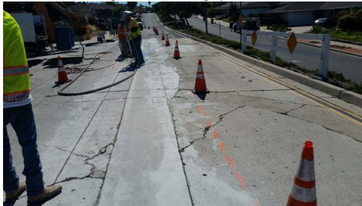
Figure 5: Saw Cutting Operations
