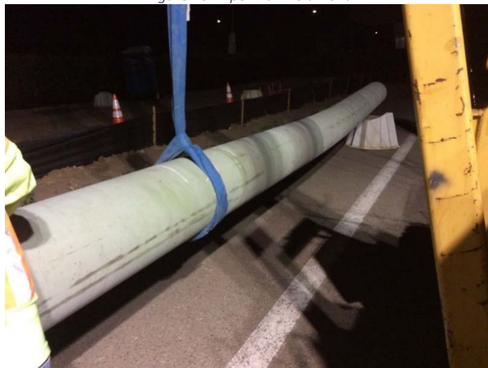
Figure 13: Pipe with Field Bend
