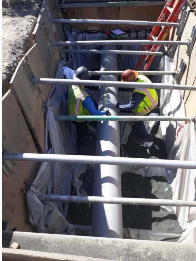
Figure 9: Bell hole inspection of Line 1600
