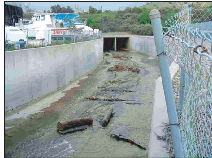
Photo 4 East of Ventura Avenue, Cañada Larga Creek has been channelized with concrete banks.
