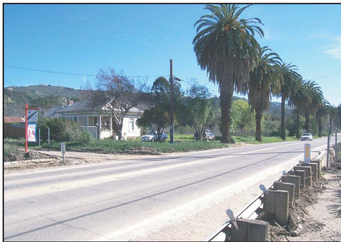
Photo 11 - North Avenue expansion area looking southeasterly from Ventura Avenue. The entire expansion area is visible to travelers on Ventura Avenue.
