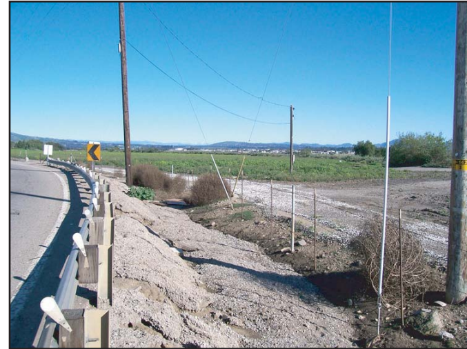
Photo 8 - Serra expansion area looking east from eastbound Bristol Road. The area south of Bristol Road fronts the Santa Clara River.
