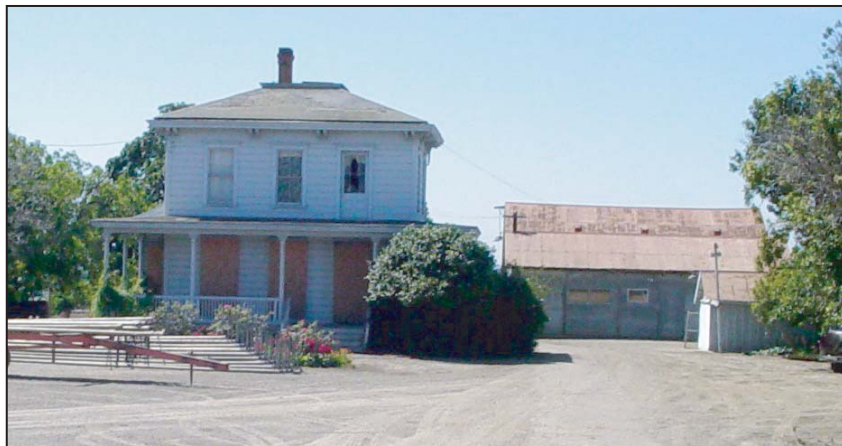
Photo 2 - Farmhouse and ancillary structures fronting Telephone Road in the Serra expansion area.
