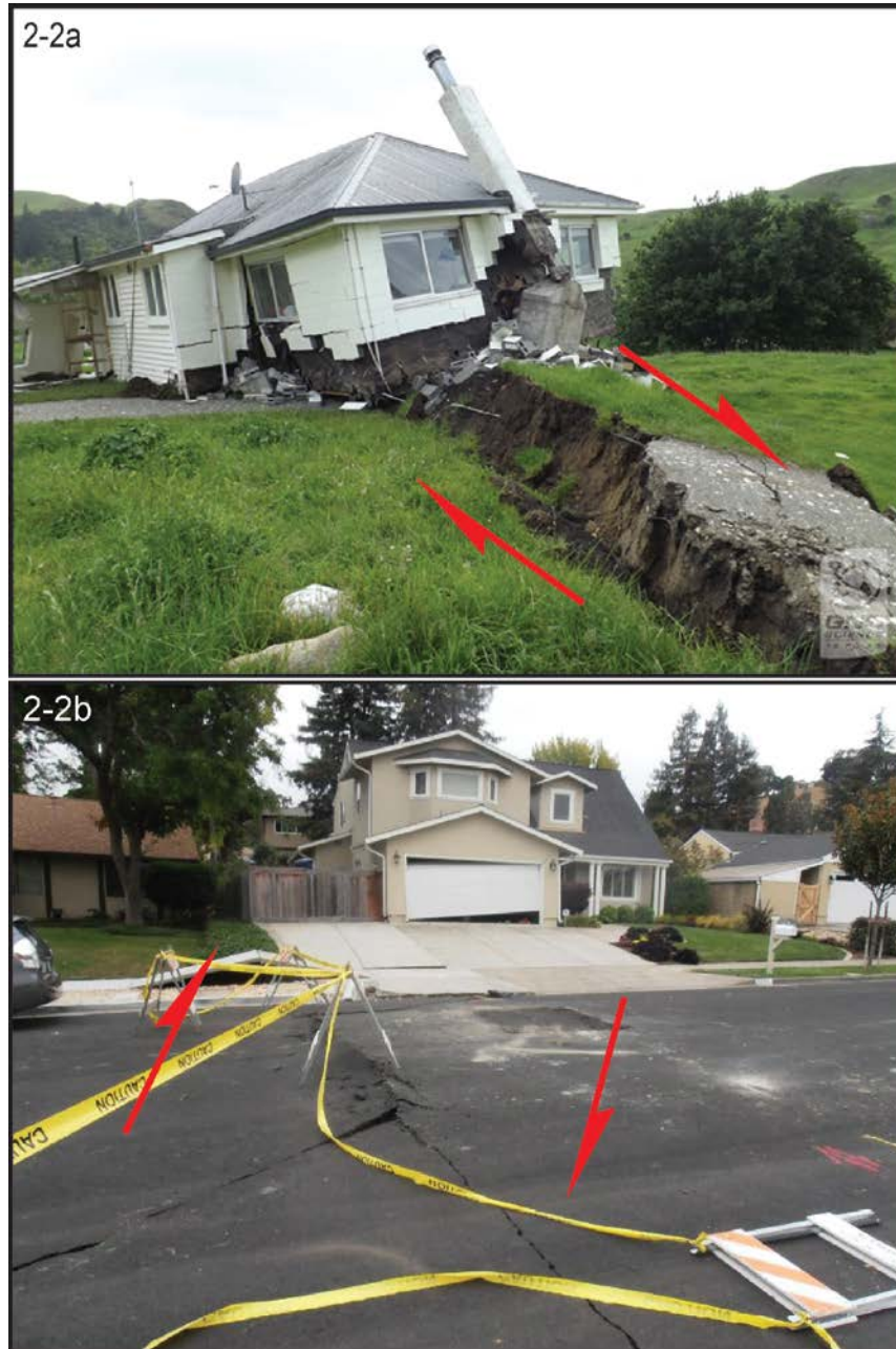
Figure 2-2a-b. 2a. Impact of surface fault rupture on a home during the November 14, 2016 M 7.8 Kaikoura earthquake, New Zealand. Fault displacement at this location was about 10 meters (33 feet) of horizontal offset. Photo credit: Pilar Villamor, GNS Science / Earthquake Commission. 2b. House damaged by surface rupture during the August 14, 2014 M 6.0 South Napa earthquake. Total displacement on the fault was less than 1 foot, yet even relatively modest amounts of fault offset required expensive (>$100,000) repairs including the replacement of the foundation of the house. Red arrows show relative trend of faulting and sense of horizontal movement.
