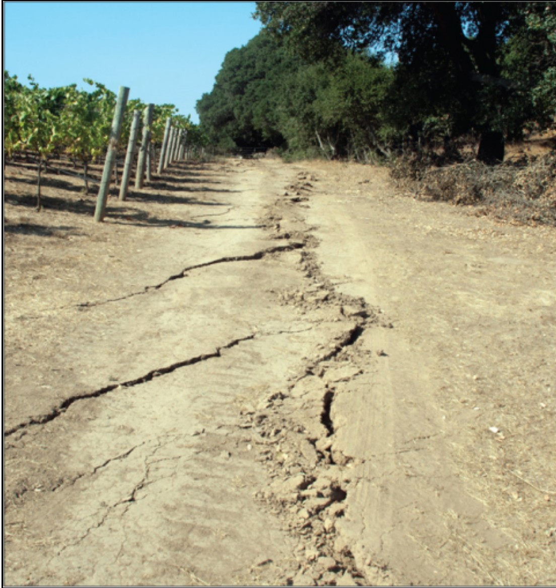
Figure 2-1. Example of surface fault rupture from the M 6.0 August 24, 2014 South Napa earthquake. Displacement at this location was about 0.5 meters (1.6 feet).
