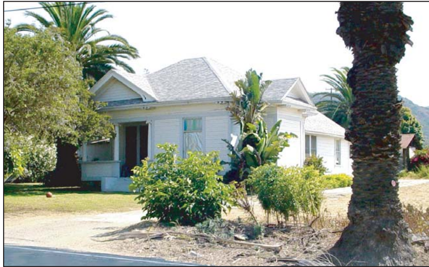
Photo 1 - Farmhouse fronting Ventura Avenue in the North Avenue expansion area.
